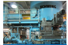
Sludge Feed Improvements
