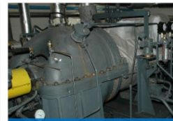
Turbine Generator Improvements
