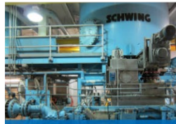
Cake Pumping Modifications
