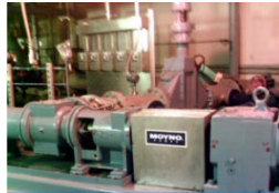
Sludge Storage Pumping Improvements
