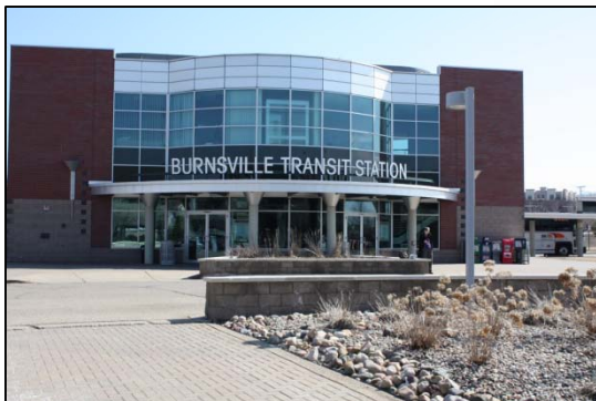
Burnsville Transit Station
