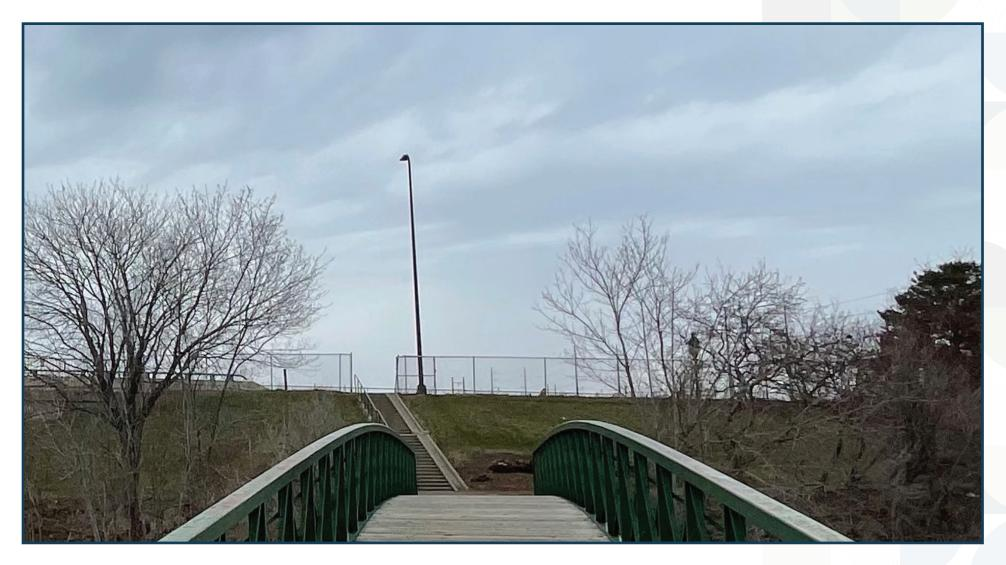
View looking north from existing marina bridge illustrating existing substandard width and non-compliant wooden deck. Proposed underpass to be constructed approximately where existing stairway is located. New accessible connections from Plymouth Avenue sidewalks and underpass/ park trails are included with the project.
