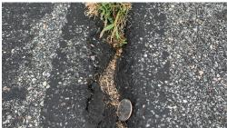
**Trail Condition:** Lateral cracks are present every 30-60 feet due to failing base material along the entire trail corridor. The pavement is no longer conducive to any pavement treatment and requires complete reconstruction to support safe and functional use for people walking, biking, and rolling.
