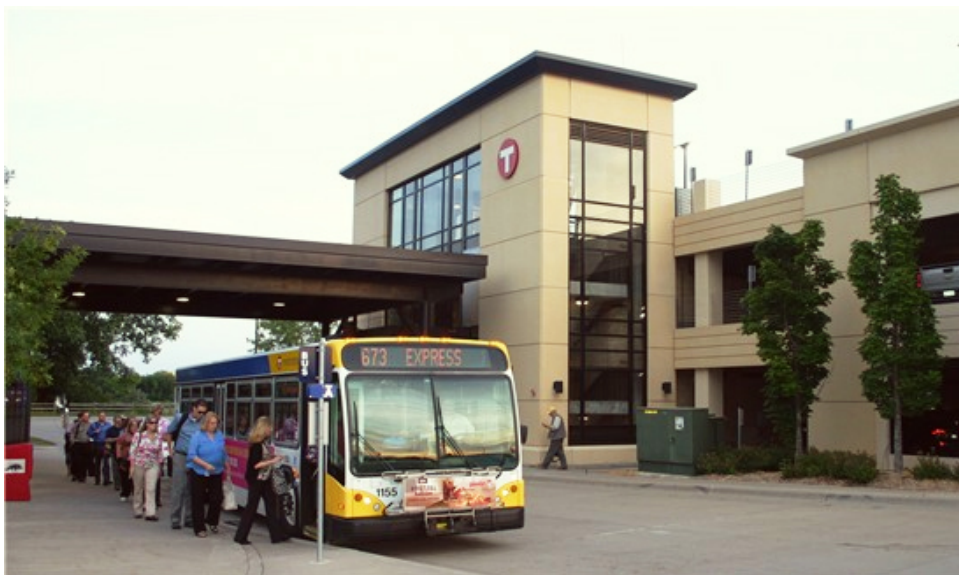
Figure 4: Offline Station, I-394 & CR 73 Park-and-Ride in Minnetonka, MN
