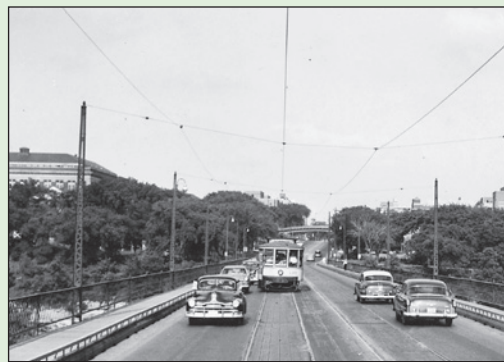
Washington Avenue bridge, by the University of Minnesota
