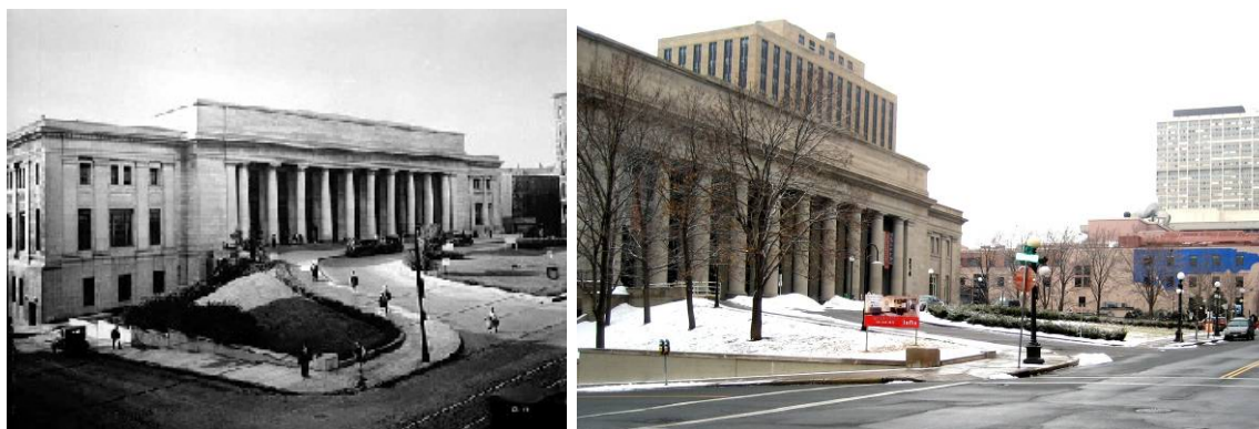
The Union Depot then and now; at left circa 1920, and at right in 2008
