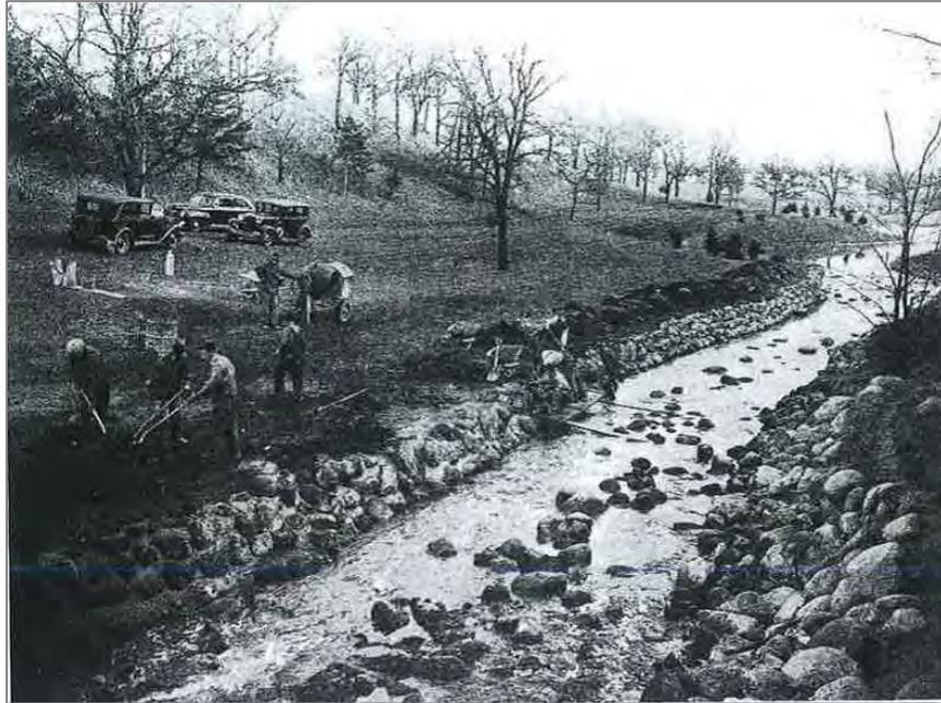
Figure 9. Federal relief workers placing riprap along Bassett Creek (MBPC 1941:33).
