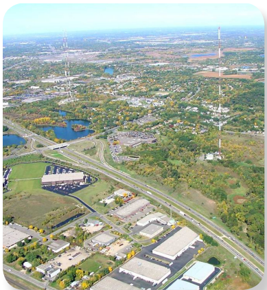
Figure 10-16: Shoreview tall tower antenna farm
