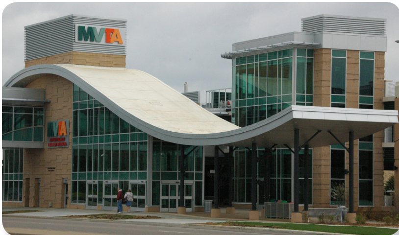
Figure 7-37: The newly constructed Apple Valley Transit station on the Cedar Avenue BRT corridor
