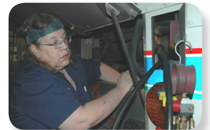
Figure 7-25: Skilled workers improve reliability of the entire system
