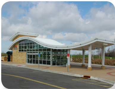
Figure 7-33: Cedar Grove Transit Station, part of Cedar Avenue BRT
