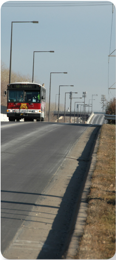
Figure 7-36: The U of M transitway is dedicated right-of-way for campus transit vehicles
