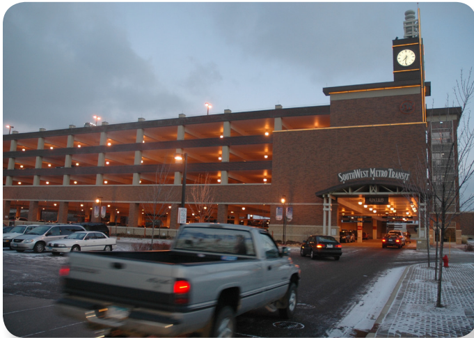
Figure 7-8: Park-and-rides concentrate trip origins in lower-density areas to create efficient express and LRT service
