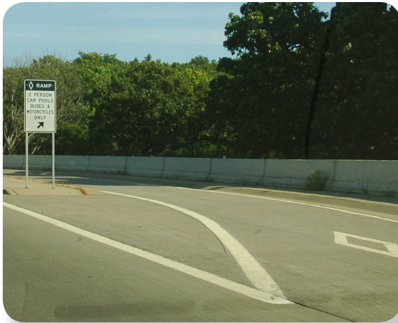
Figure 7-27: Ramp meter bypasses are transit advantages that encourage ridership by improving transit time.
