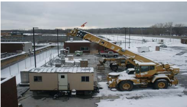
Construction of the Metro Plant disposal site is nearly complete.
