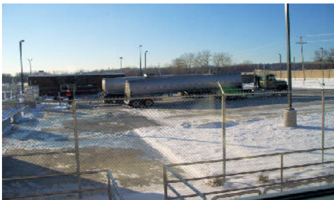
Trucks discharging their loads at Metro LWR
