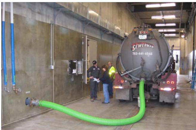
One of two discharge ports at Fridley LWR
