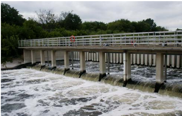
Metropolitan Wastewater Treatment Plant effluent channel
