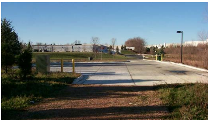
Pictured above is the Chanhassen liquid waste hauler disposal site. This site will need to be upgraded according to the proposed plan requirements.
