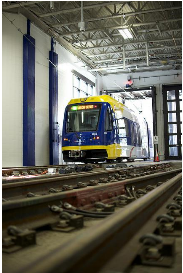
Lowertown Operations & Maintenance Facility, St. Paul. Source: Metro Transit Flickr account: https://www.flickr.com/photos/metrotransitm/
