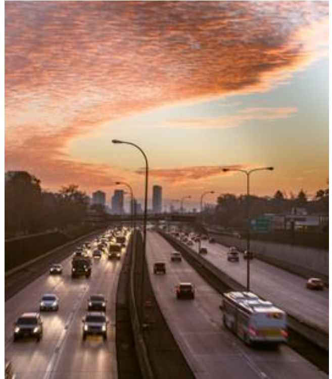
I35W North. Source: Metropolitan Council Digital Image Library
