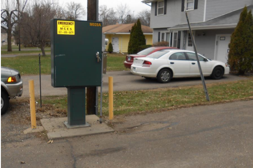
Meter RTU/PLC cabinet raised 3 ft and inside the meter RTU/PLC cabinet. Source: Metropolitan Council Digital Image Library
