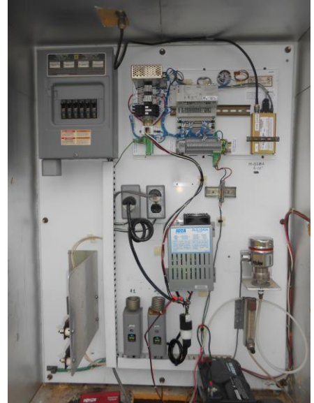
Meter RTU/PLC cabinet raised 3 ft and inside the meter RTU/PLC cabinet. Source: Metropolitan Council Digital Image Library
