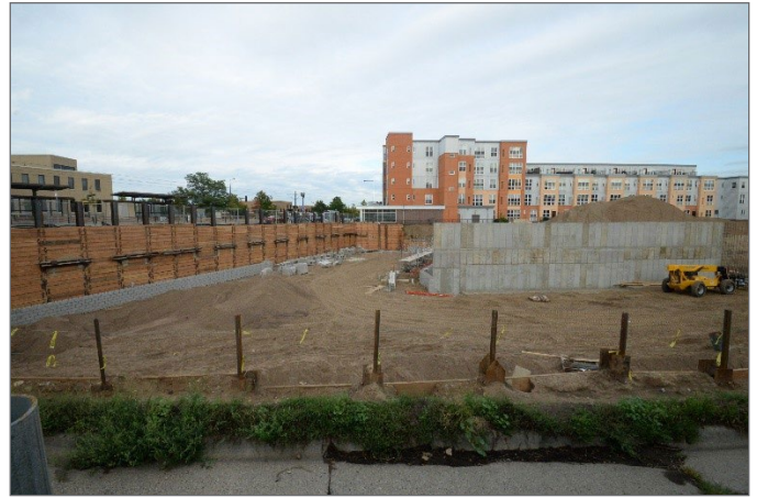
Construction underway on 2700 University Ave. Source: Metropolitan Council
