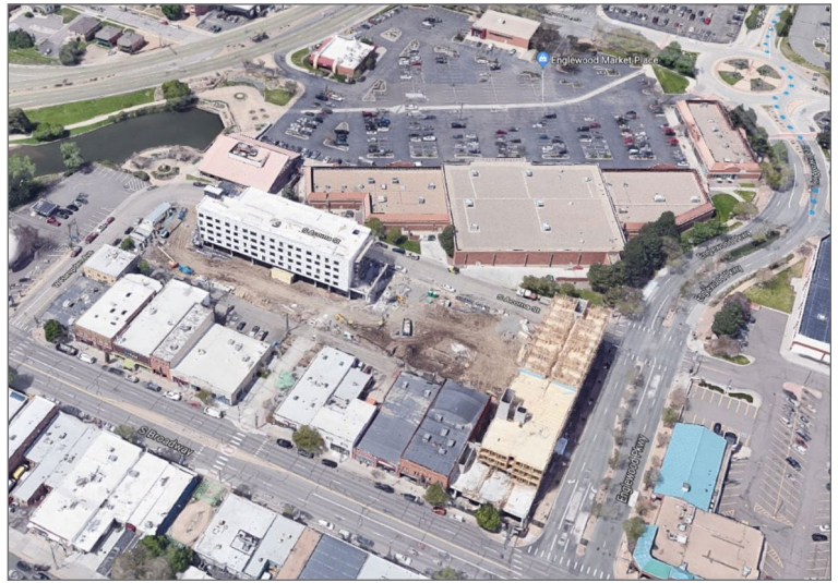
Looking west from South Broadway Street toward the lower-density retail uses in CityCenter . Under construction are the Broadway Lofts (right, foreground) and Acoma Lofts (left, middle ground), 111 units of affordable housing. Potential daylighting of Little Dry Creek could occur in the area currently occupied by the large amount of surface parking.
