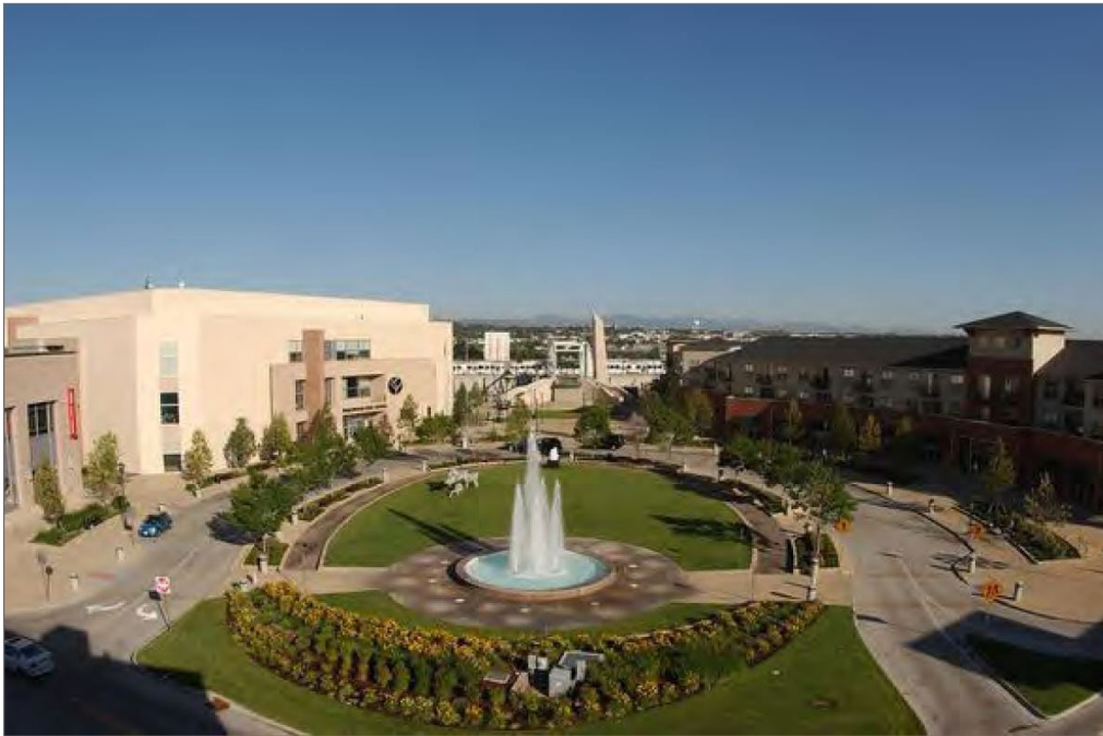
CityCenter Englewood. Looking west toward Englewood Station in the distance with Englewood Civic Center to the left. (Photo courtesy City of Englewood.)
