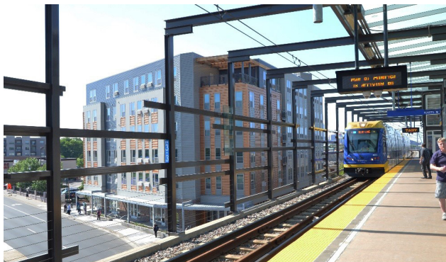
Minneapolis. View from Lake Street/Midtown Station platform looking northwest toward project.
