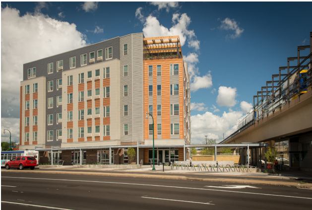
Looking northwest across Lake Street west of METRO Blue Line.
