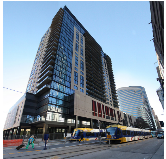
Downtown Minneapolis, METRO Green Line / Blue Line Nicollet Mall Station. High-density mixed-use development integrates into the station, “raising the bar” for TOD.
