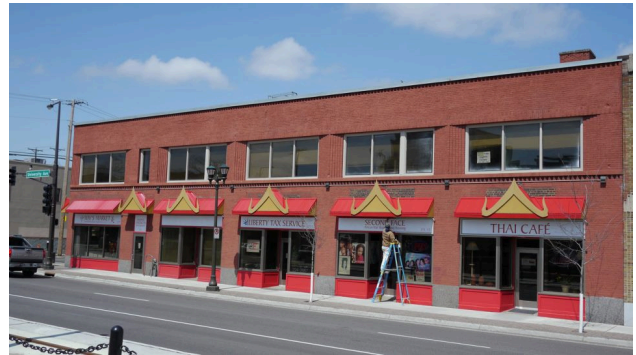
New façade of May's Market, at the corner of University and Western Avenues, incorporating the “Little Mekong” theme for the station area.
