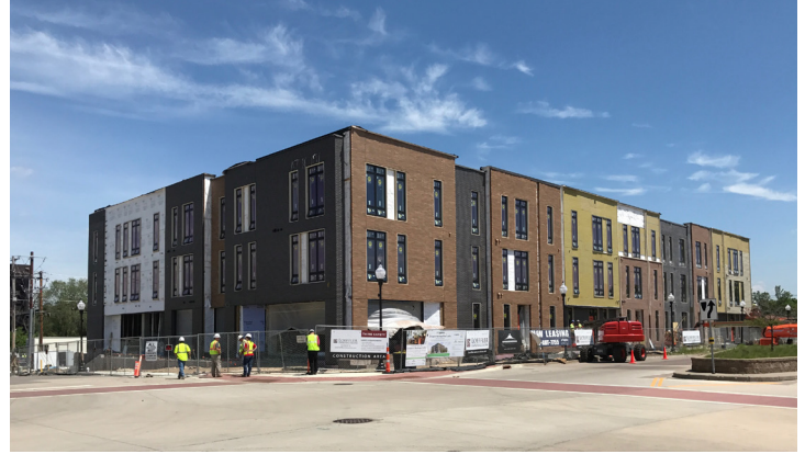
After (Near Completion)
