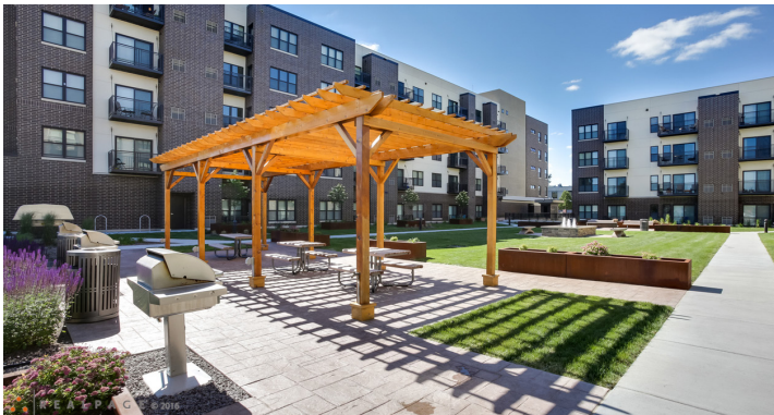
Gallery Flats includes a landscaped plaza on top of underground parking
