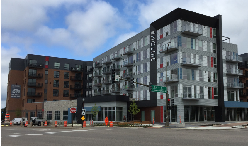
The Moline, a 241-unit luxury apartment complex across from the LRT station
