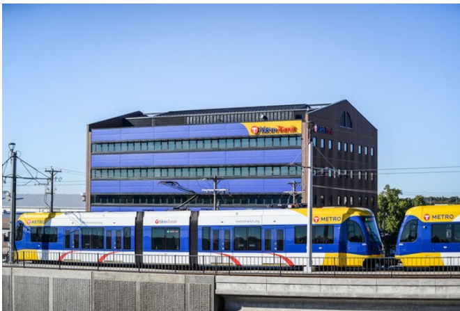
A Green Line train passes by the Heywood Metro Transit building in Minneapolis.
