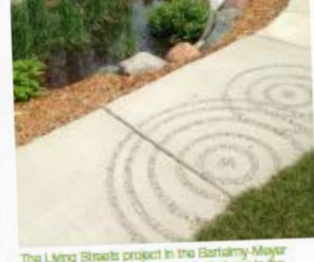
The Living Streets project in the Bartelmy-Meyer Neighborhood includes etched raindrops in the sidewalk adjacent to each rain garden.
