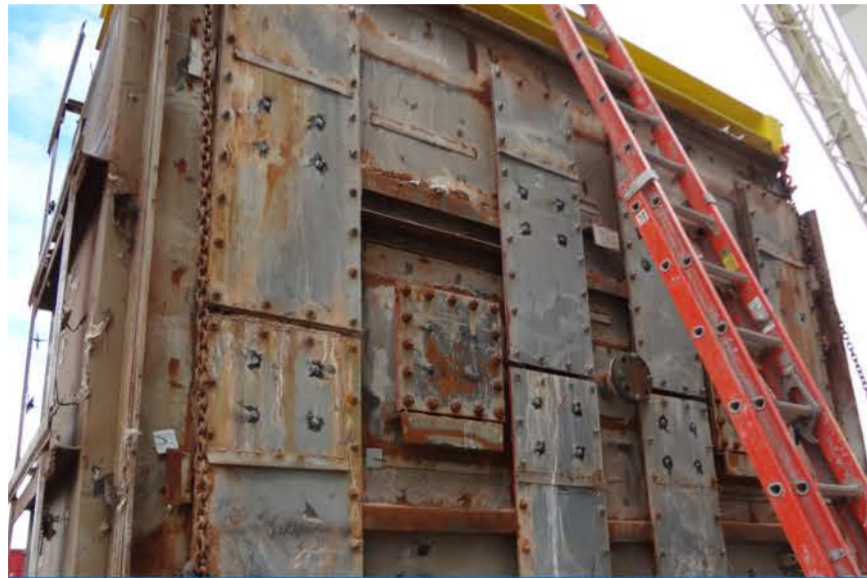
WHB Economizer Replacement
