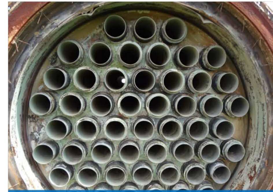
Primary Heat Exchanger Replacement
