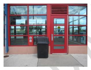
The photo to the left is an example of a simple fix that requires Metro Transit public facilities staff to relocate the receptacle to make the power-assisted door functional.
