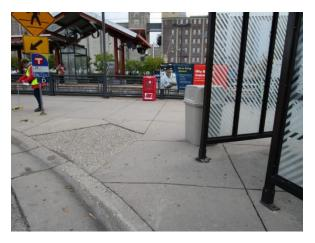
The picture to the left shows a cross slope of 8.1% (above the 1:48 threshold required by ANSI 403.3). This is an example of a complicated fix since the bus shelter is connected to heat and light and cannot be easily relocated.
