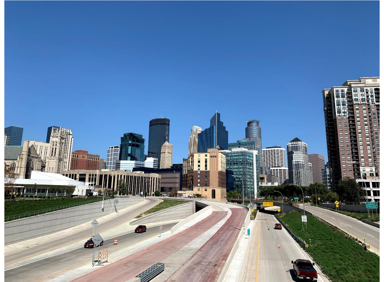
12 th Street Bus-Only Ramp into Downtown Minneapolis
