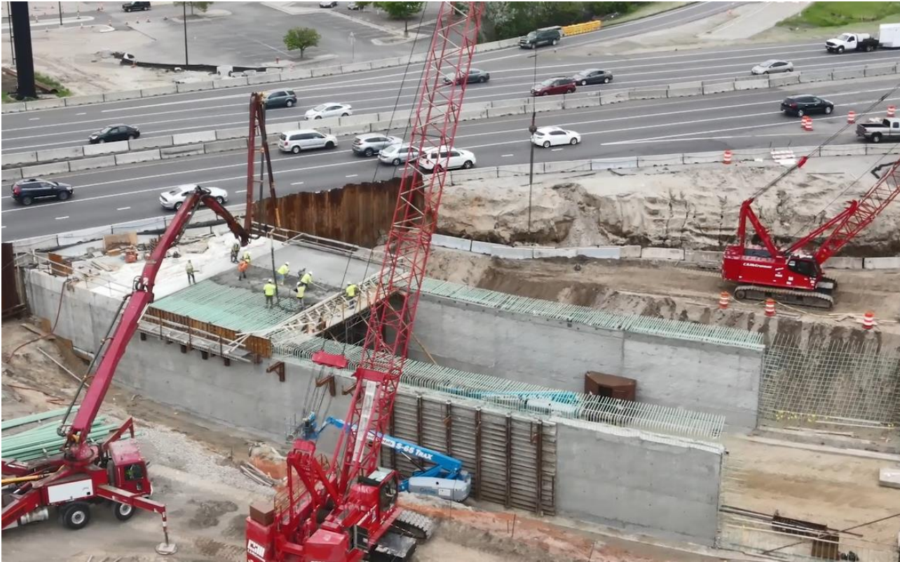
Structure Construction May 2021
