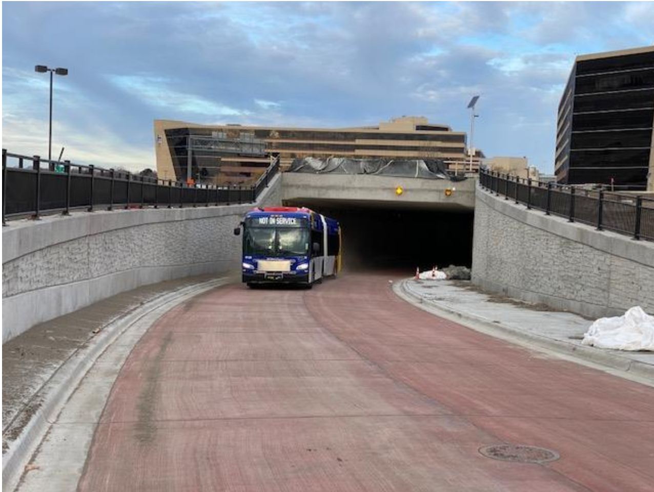
Bus Testing in the Knox Avenue Tunnel
