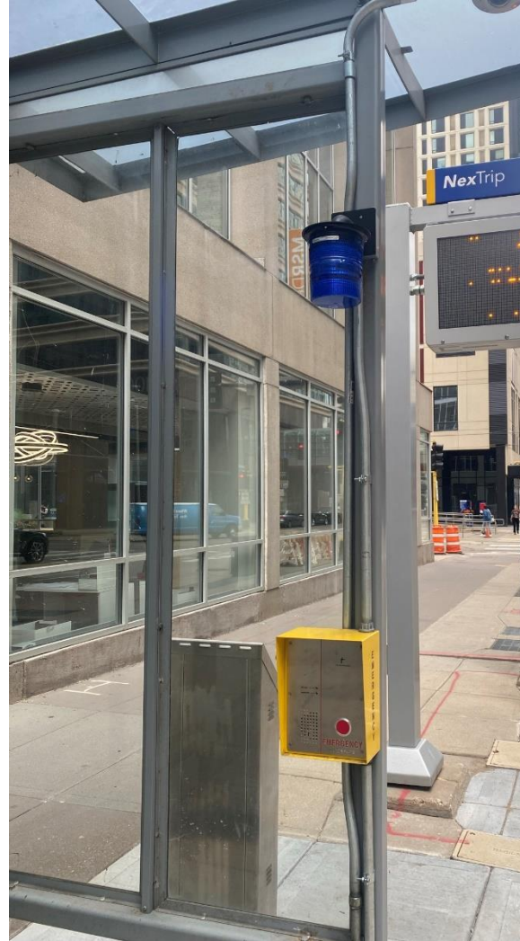
In-Progress Station Modifications
