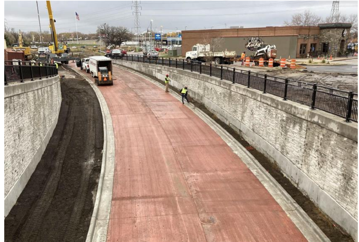
Guideway Construction Late 2021
