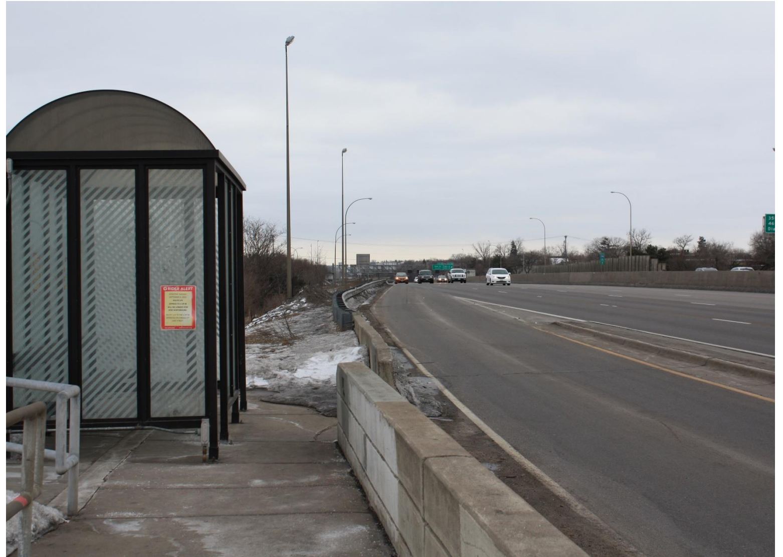
Previous Bus Stop on Freeway Shoulder
