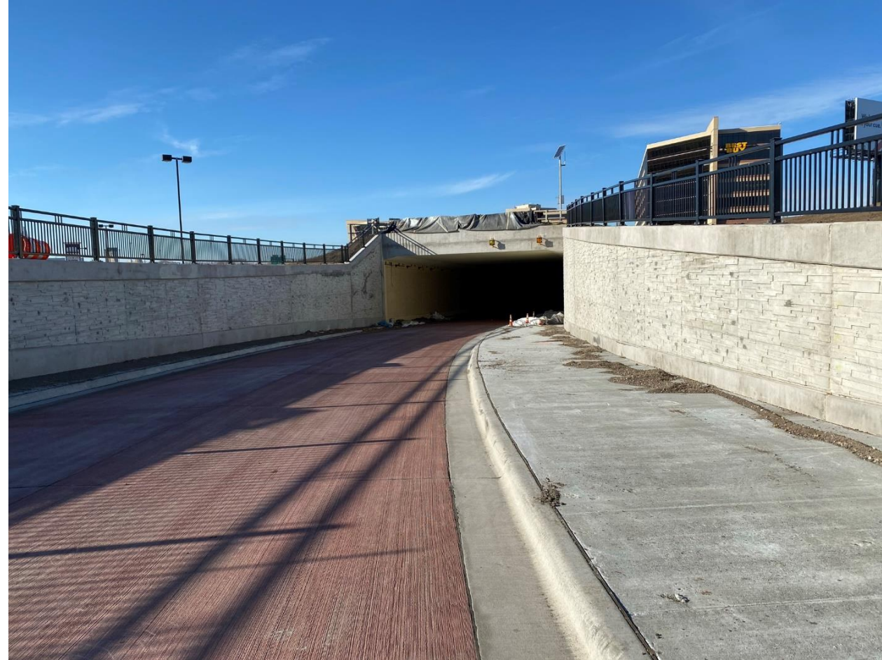
Northbound Tunnel Portal
