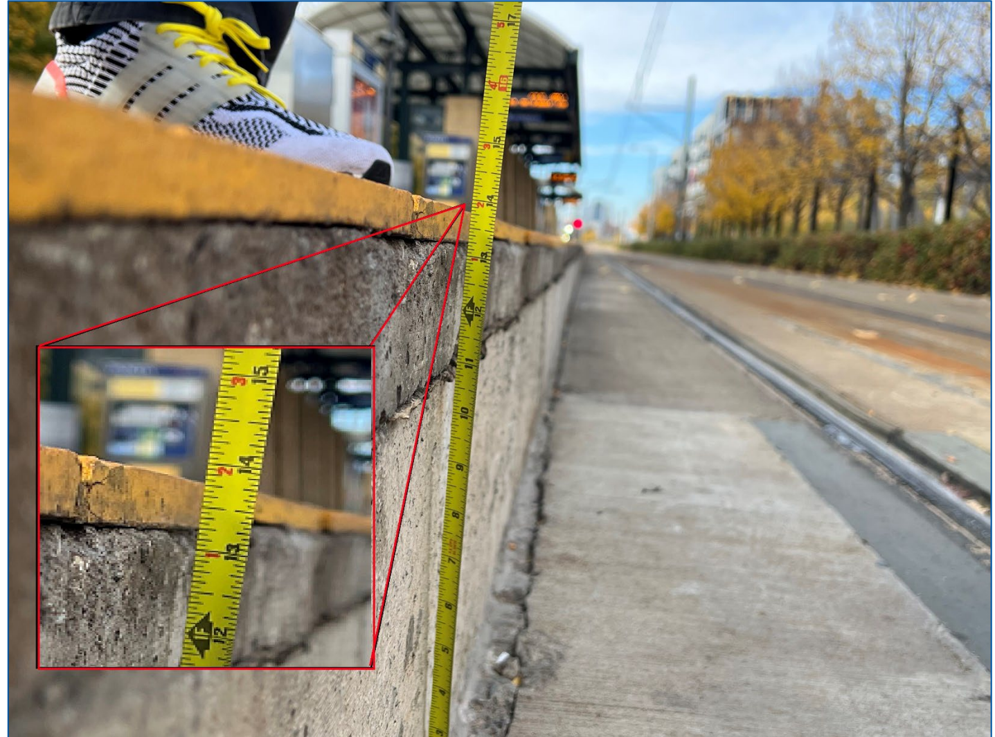
Bloomington Central Station, METRO Blue Line
