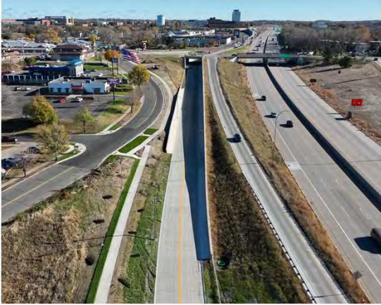
BRT Guideway underpass at Ruth St
