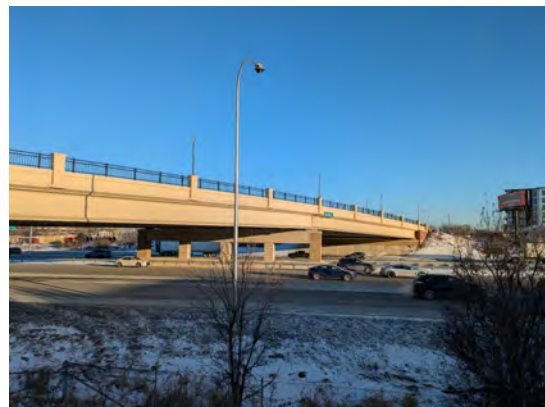
BRT Bridge at Bielenberg
