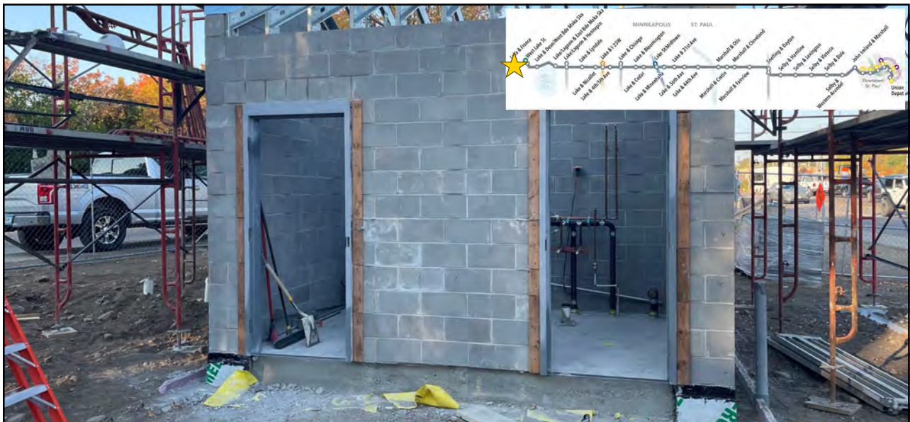
Lake & France – operator restroom facility October 2024
