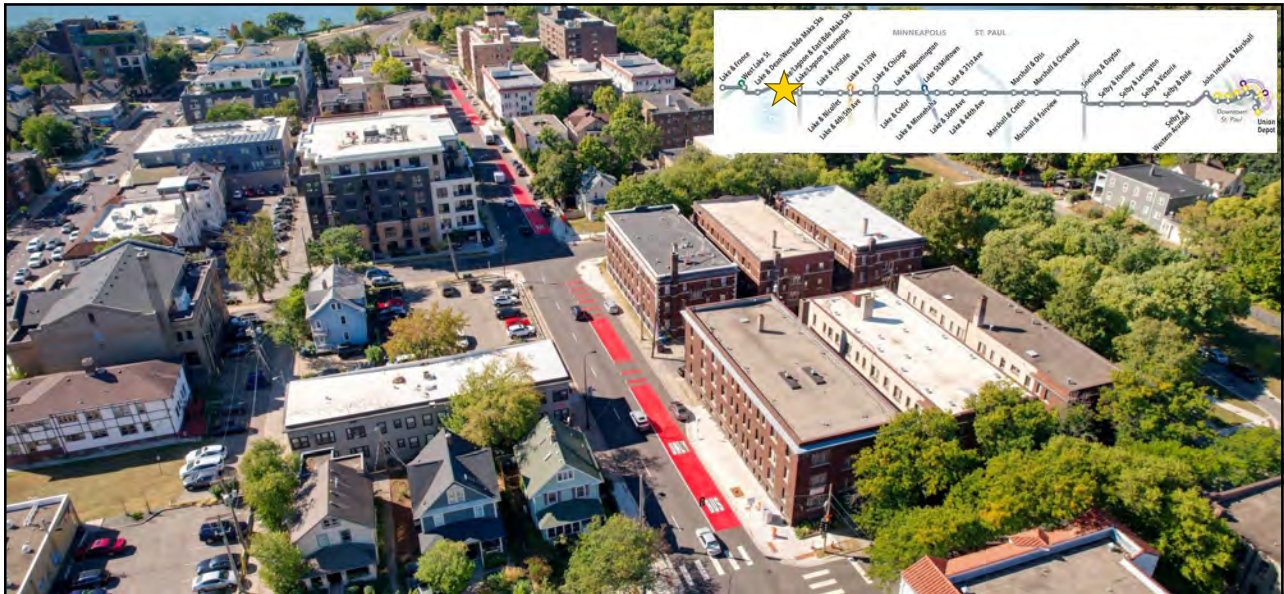
Lagoon Avenue local improvements September 2024
