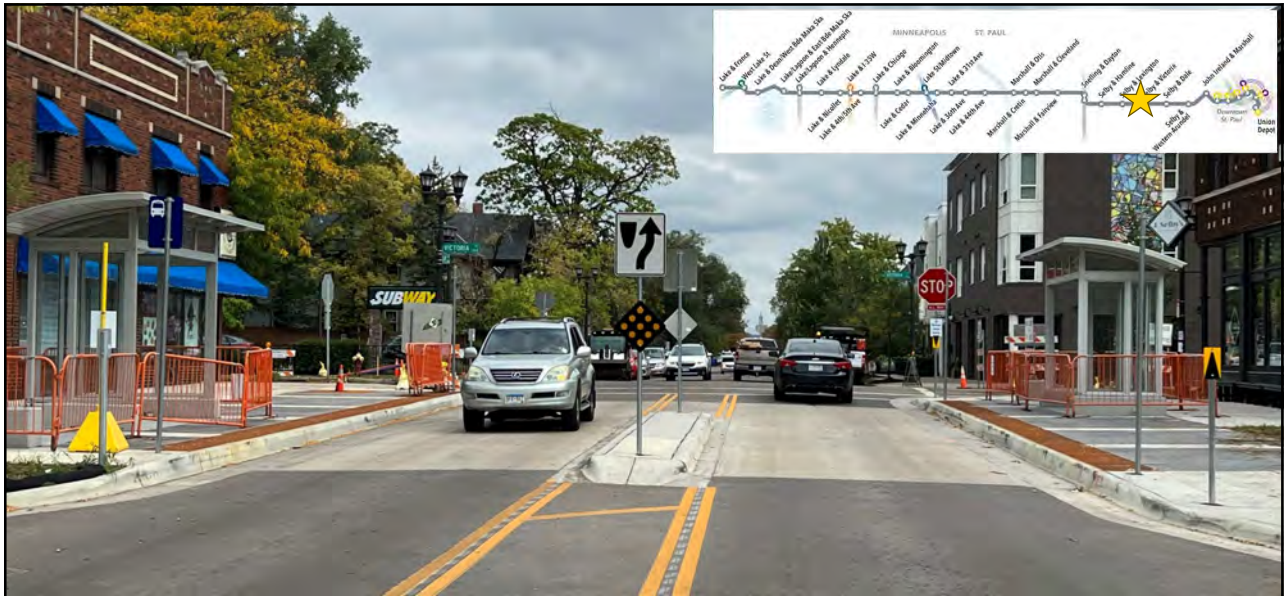
Selby & Victoria – both platforms September 2023
