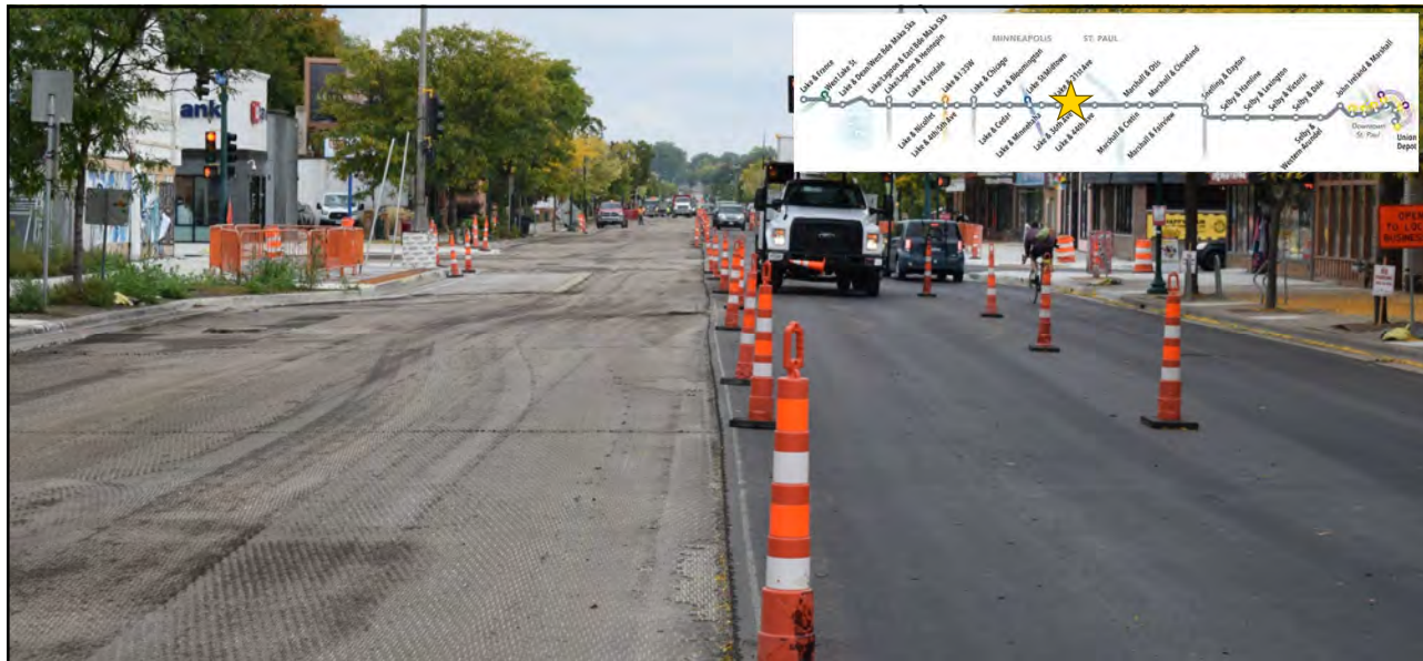
Lake Street local improvements – mill & overlay September 2023
