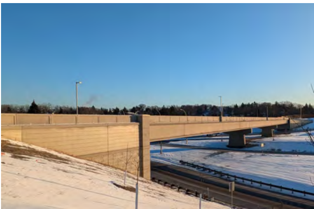
BRT Guideway at Etna
