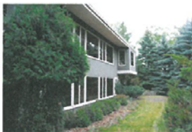
Former Wallo house.
