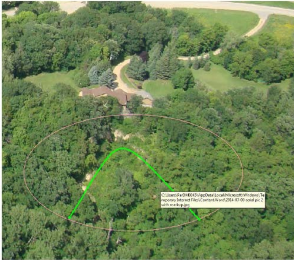
Photo 2 View of Slide Area with House in the Background Looking Squarely at Face of Scarp
