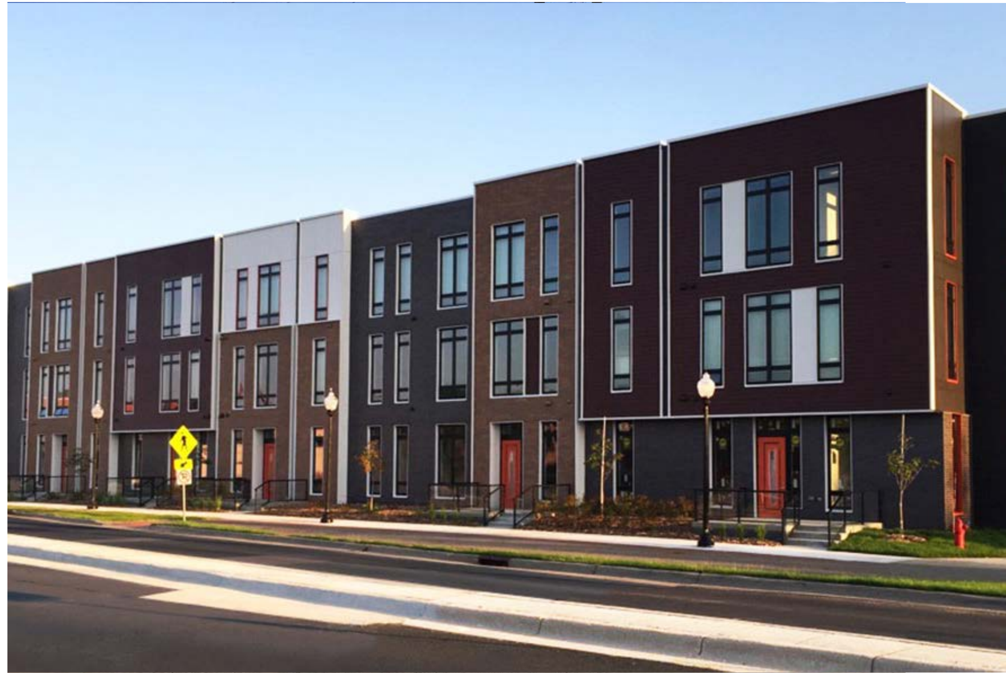
Artspace Hastings River Lofts, Hastings
