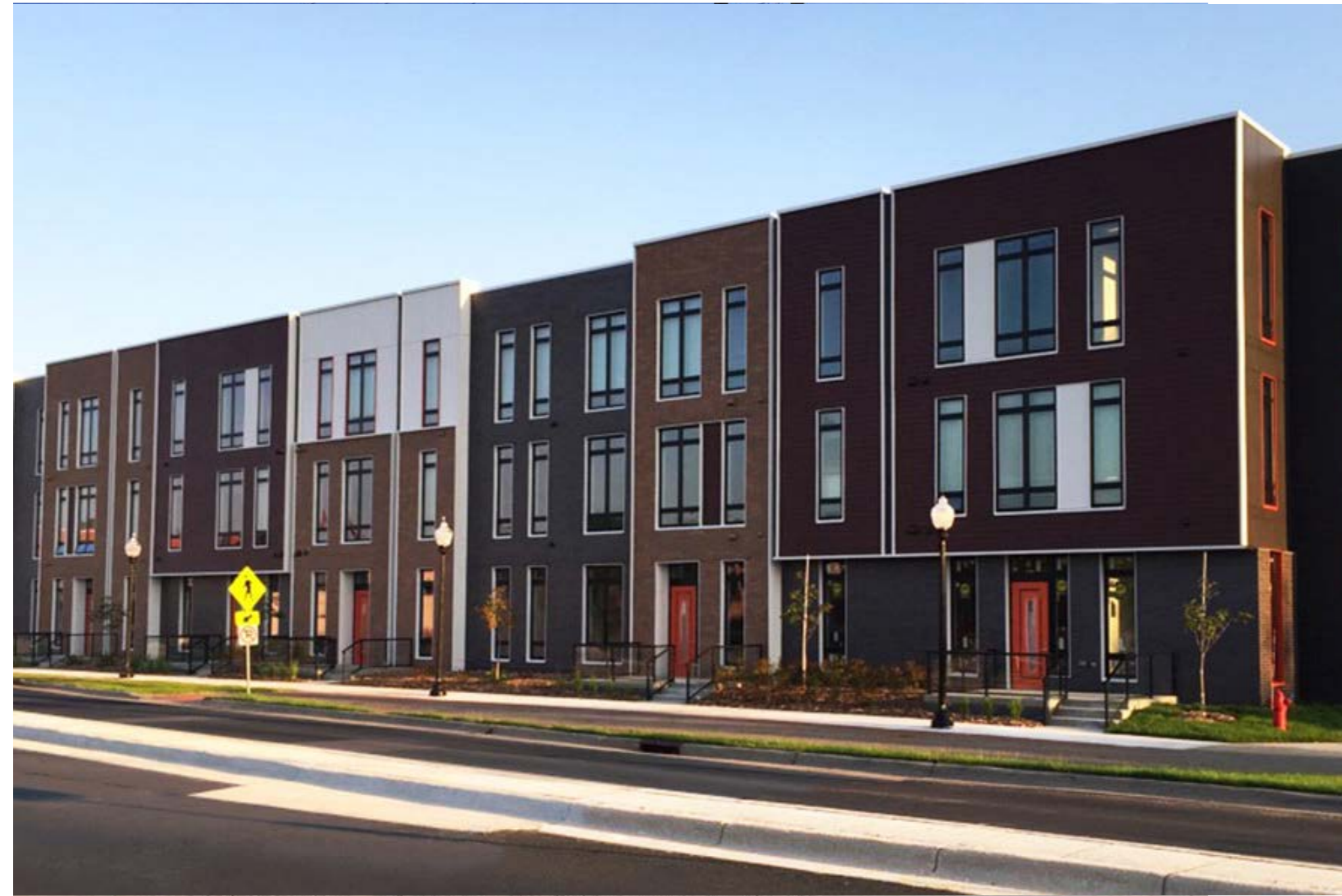
Artspace Hastings River Lofts, Hastings
