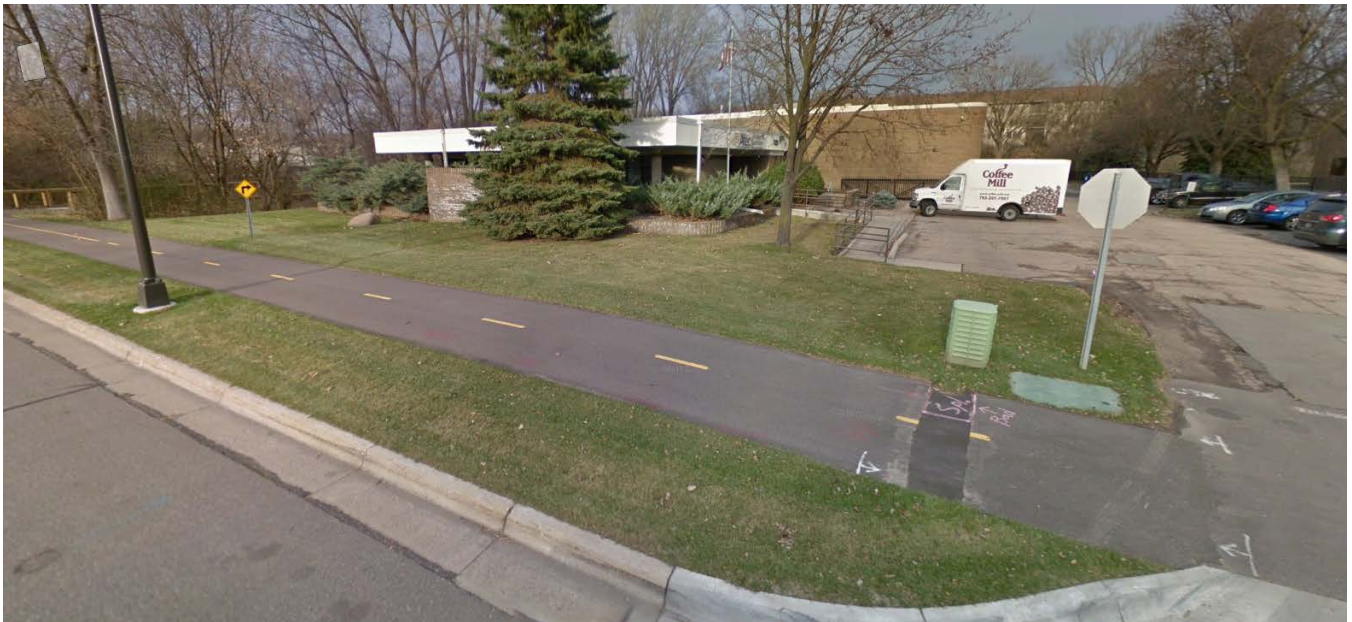
Figure 3. Google image of subject parcel showing completed trail.
