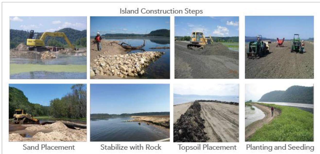
Figure 4: Island Construction Steps (MPA pg. 6)
