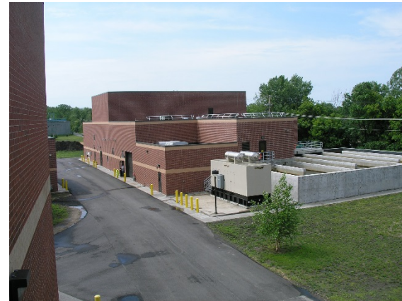
Mankato Water Reclamation Plant
