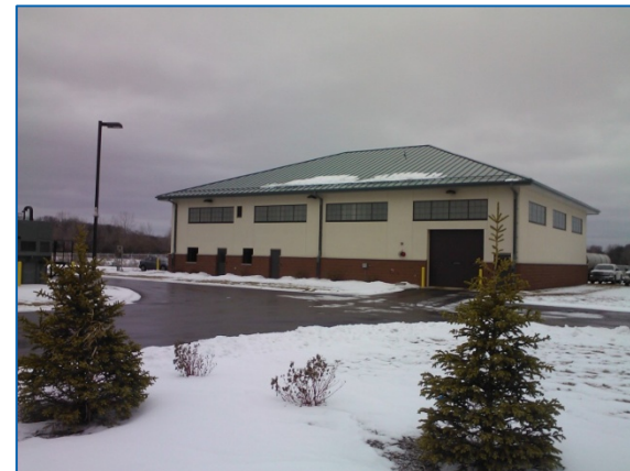
East Bethel Water Reclamation Facility
