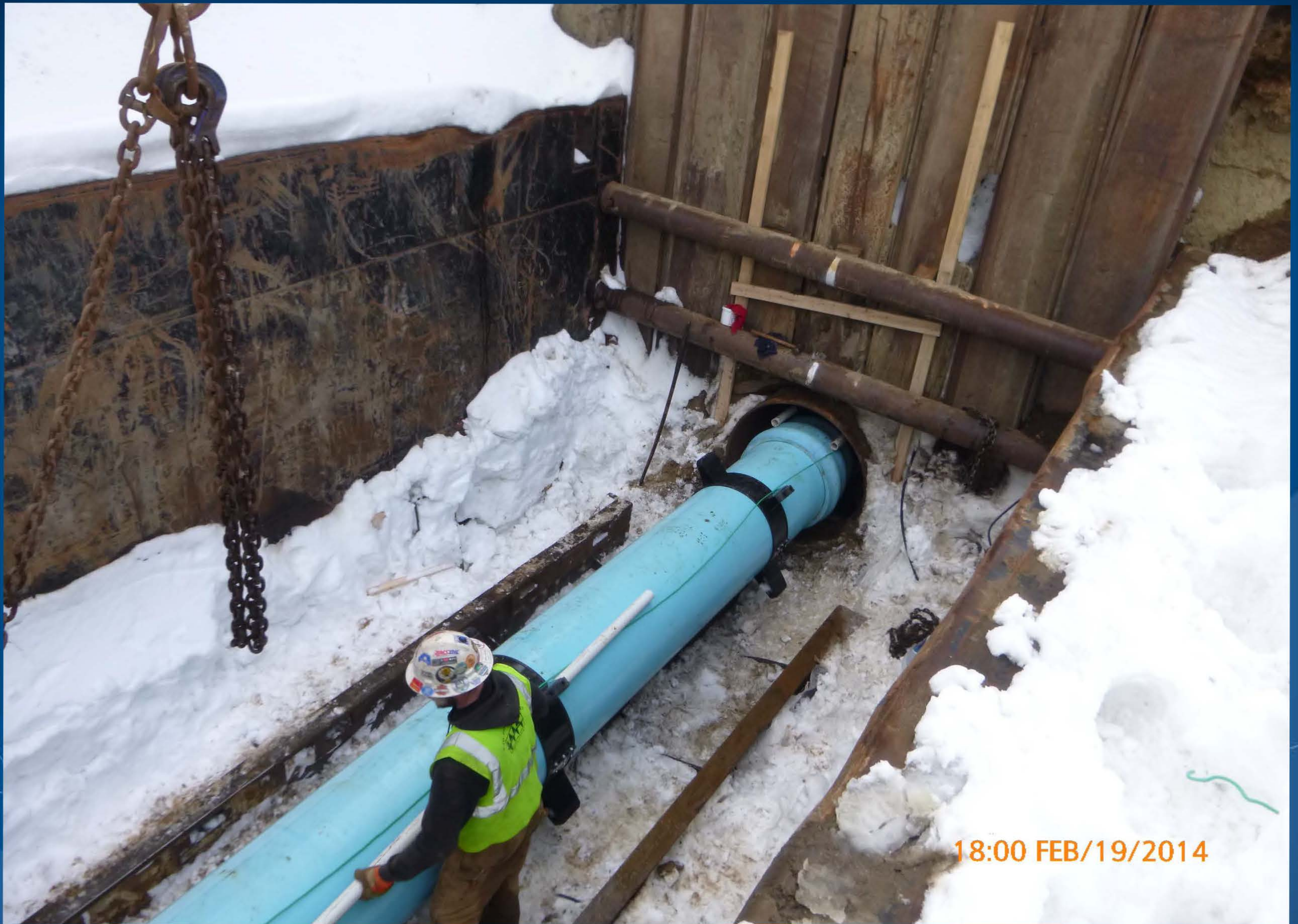
Excelsior Lift Station L19 Forcemain Jacking
