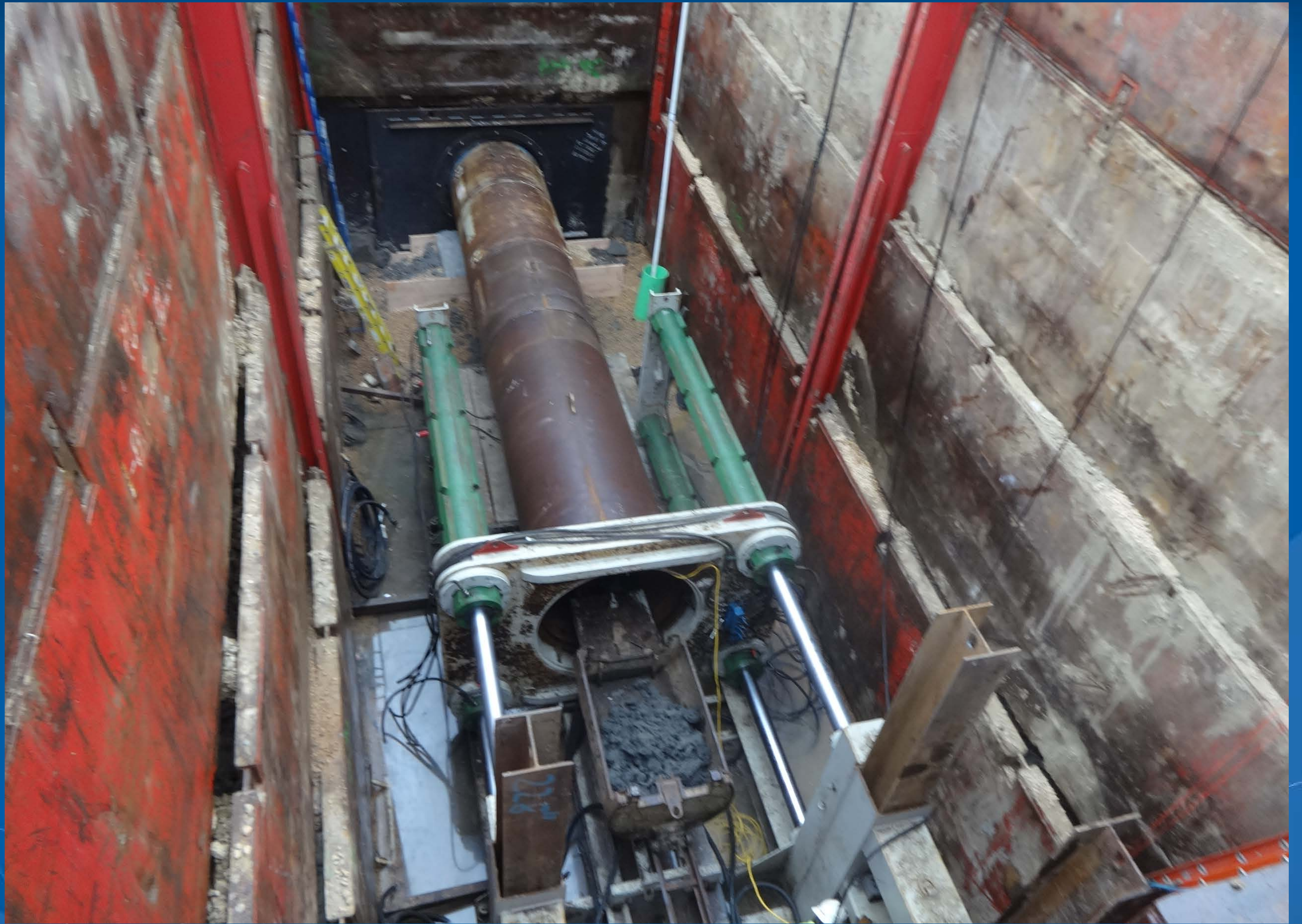
Mound Interceptor 6-MO-650 Jacked Tunnel Casing for 36-inch Gravity Sewer
