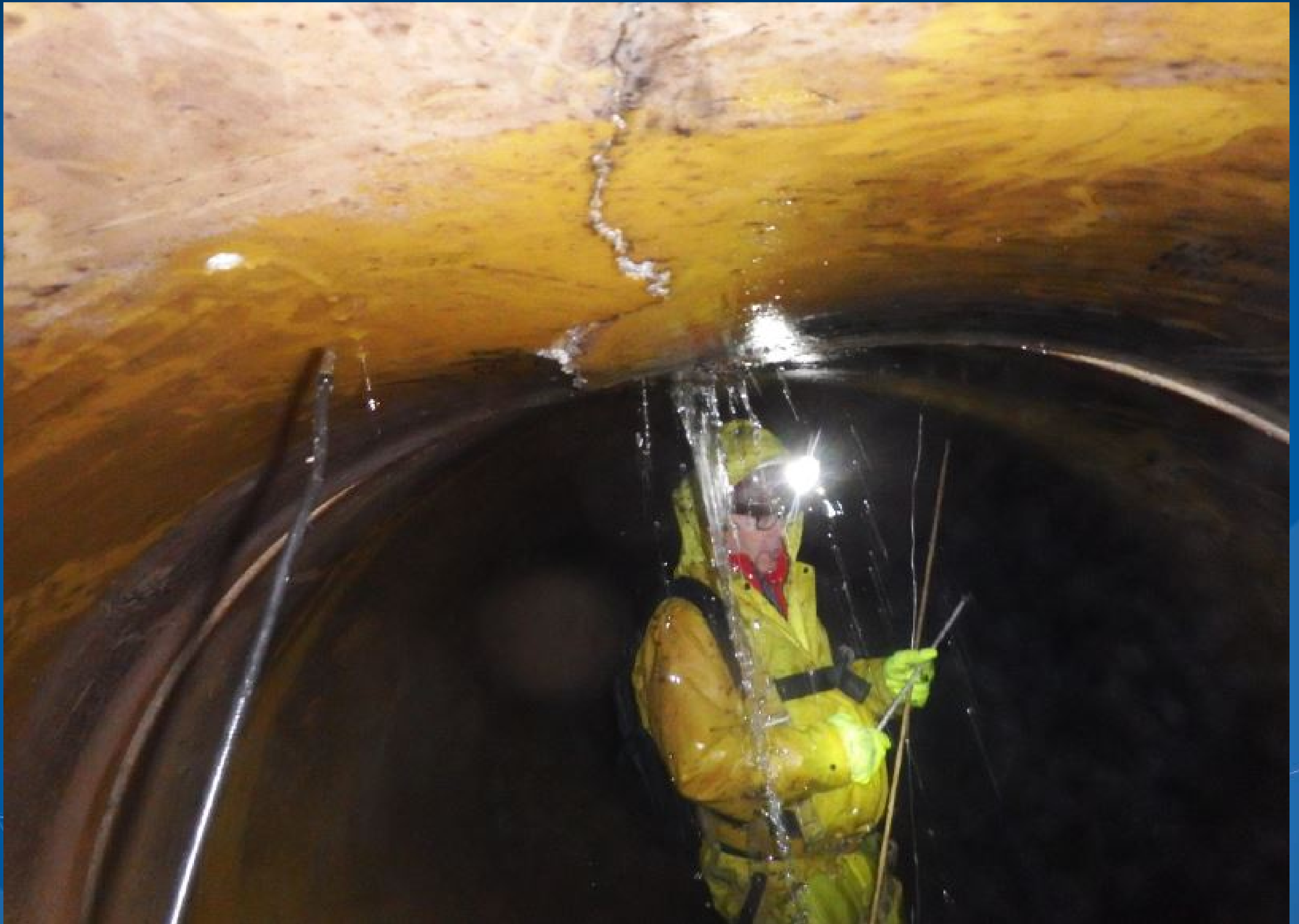
Woodbury 9701 Tunnel Interceptor Inspection and Evaluation
