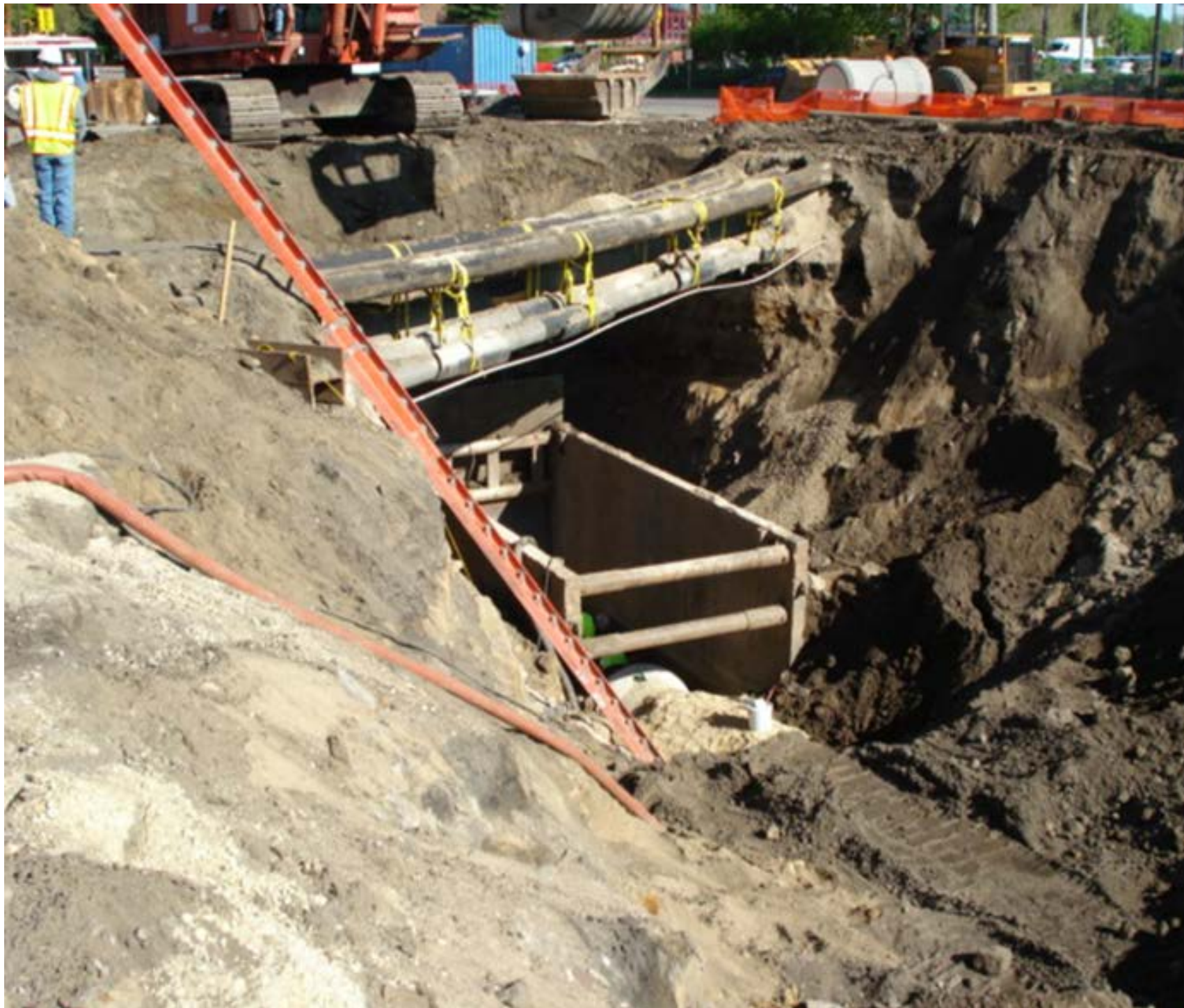
Open cut west of MH5
