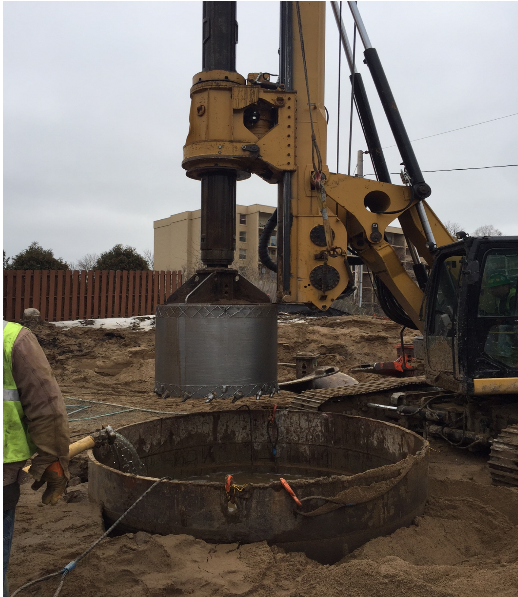
Excavating soil from inside a 72\"/>
