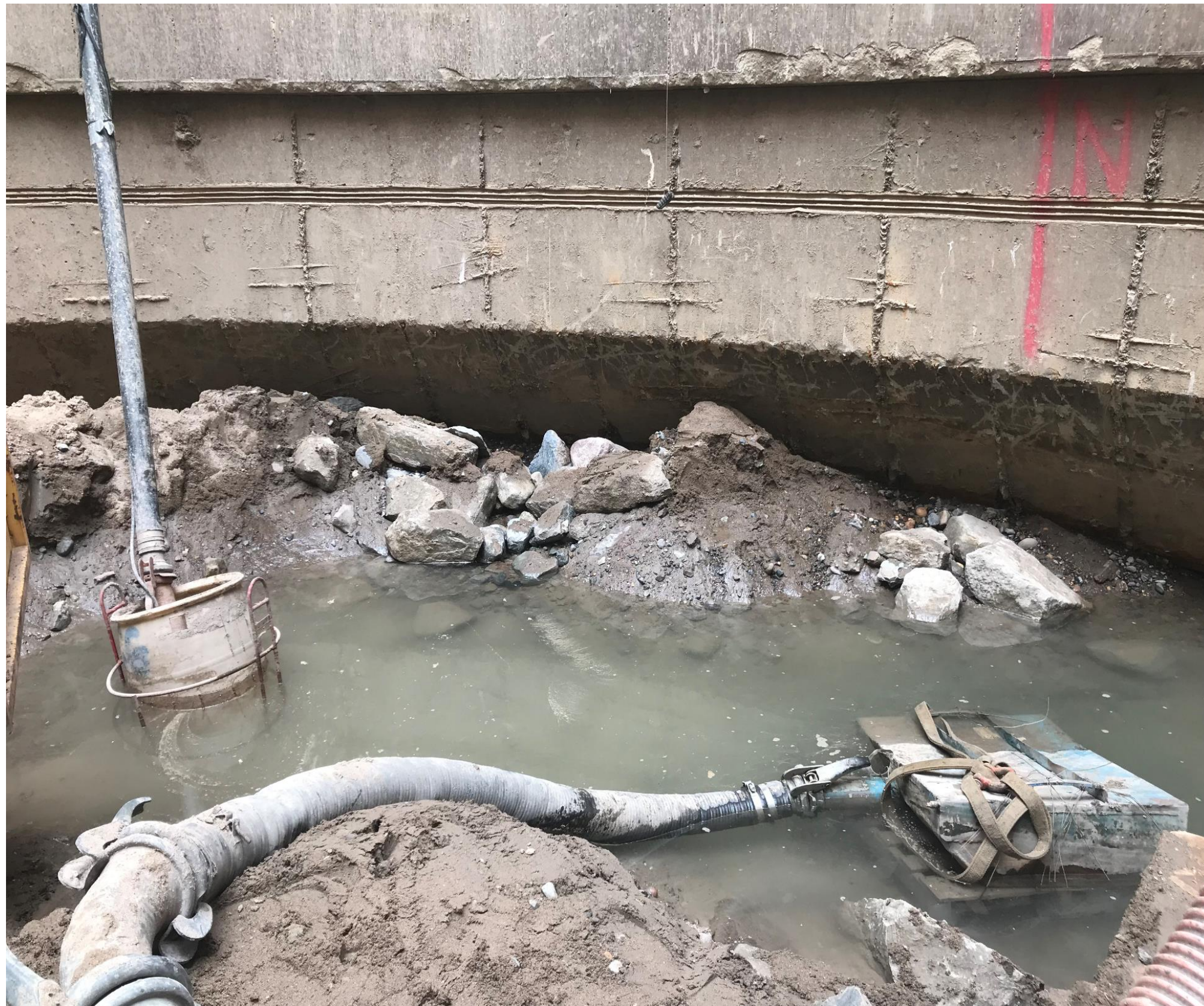
Groundwater inside the caisson
