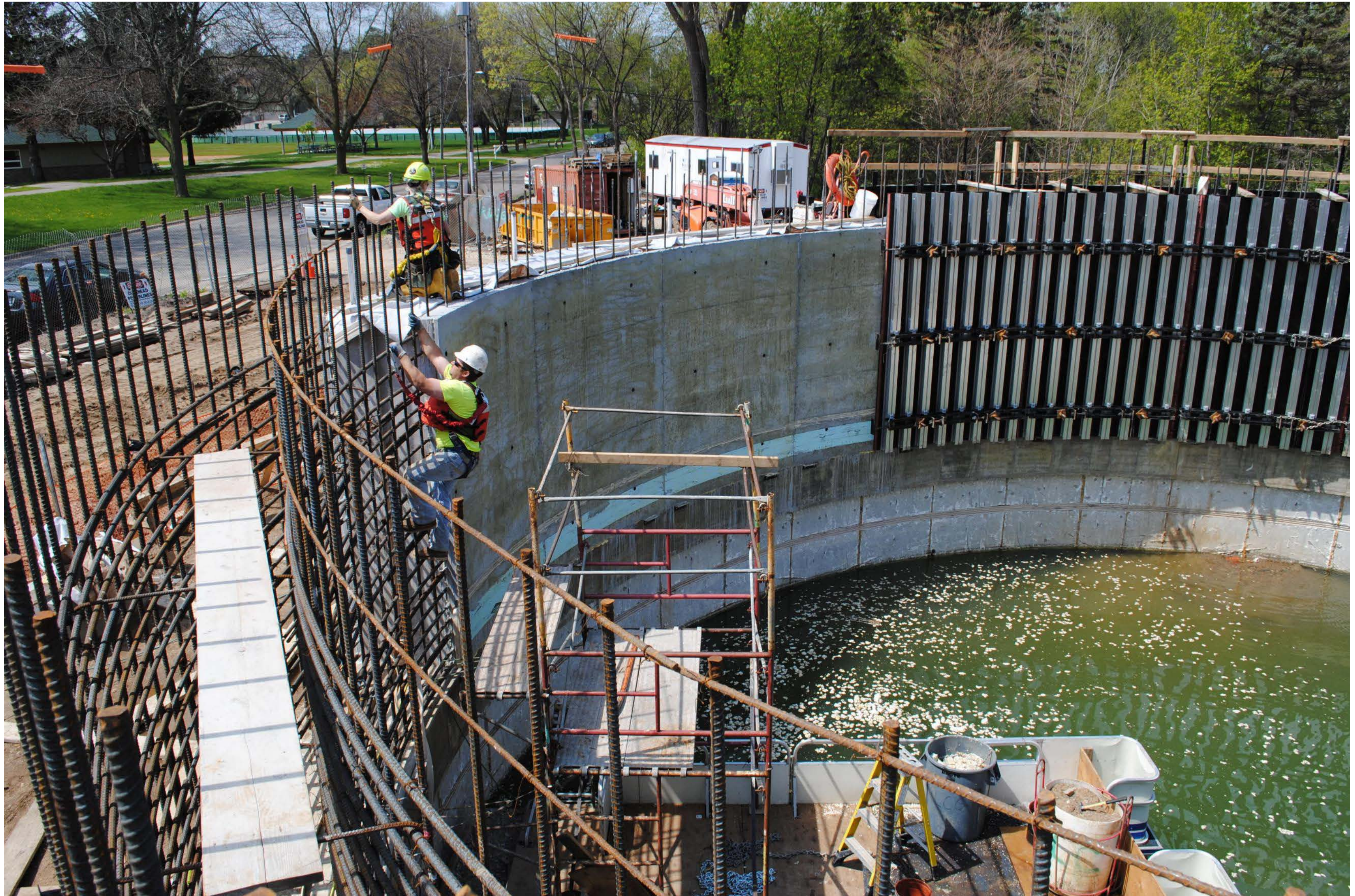
Ring Construction in Progress
