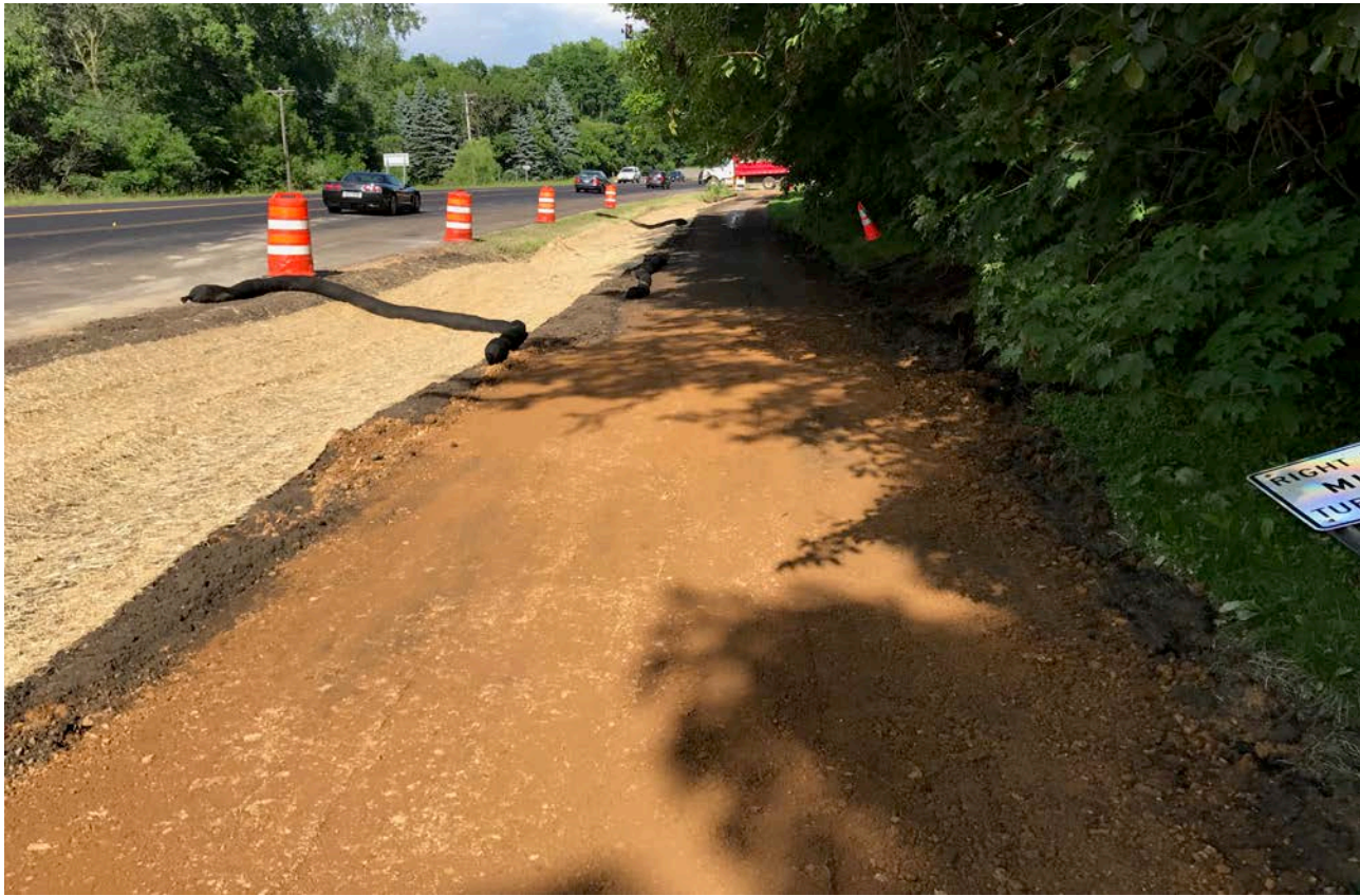
Restoration and temporary trail reconstruction following repair
