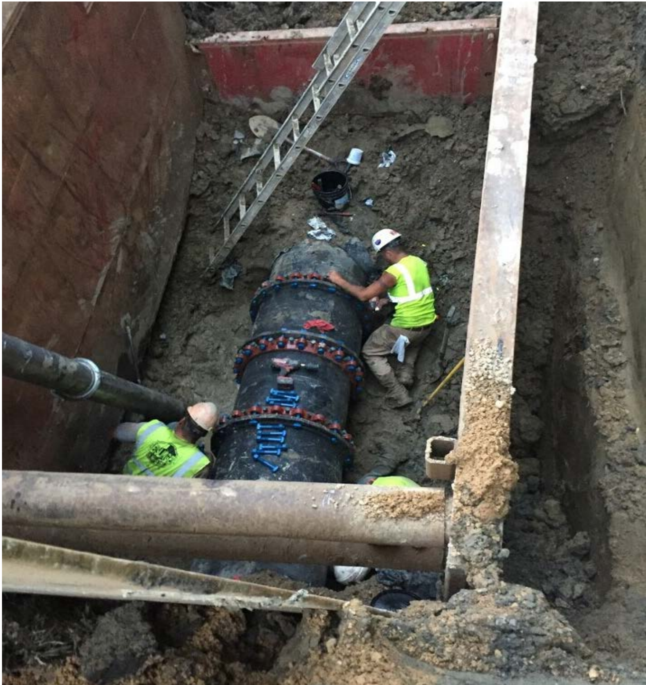
New pipe and fittings being installed at repair site
