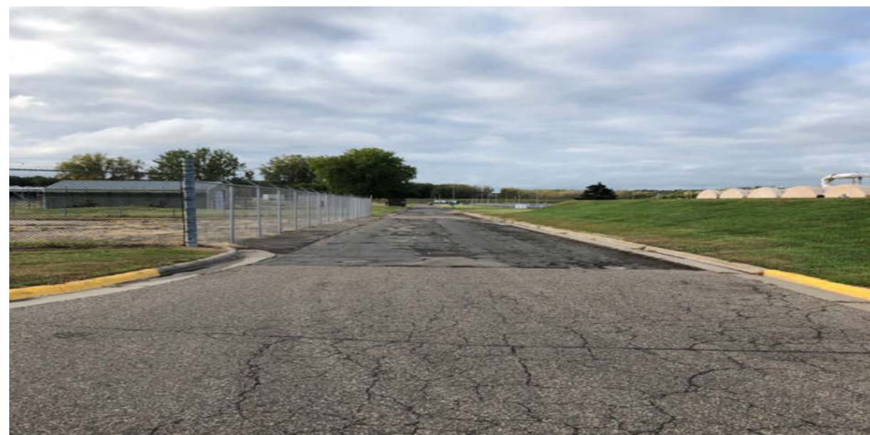
Current condition of 6 th street
