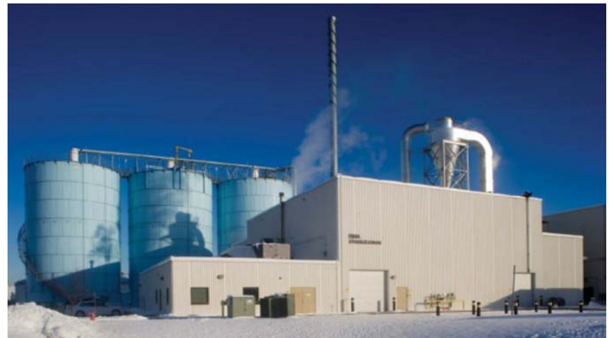
Final Stabilization Facility
