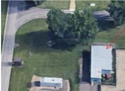
Substation Building Rehab Phase 3
