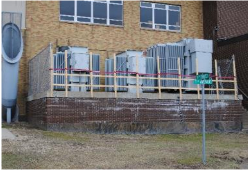
Transformer Upgrade Phase 1
