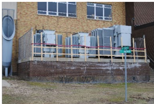
Transformer Upgrade Phase 1
