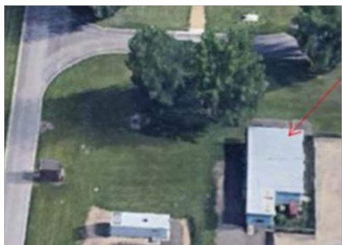
Substation Building Rehab Phase 3
