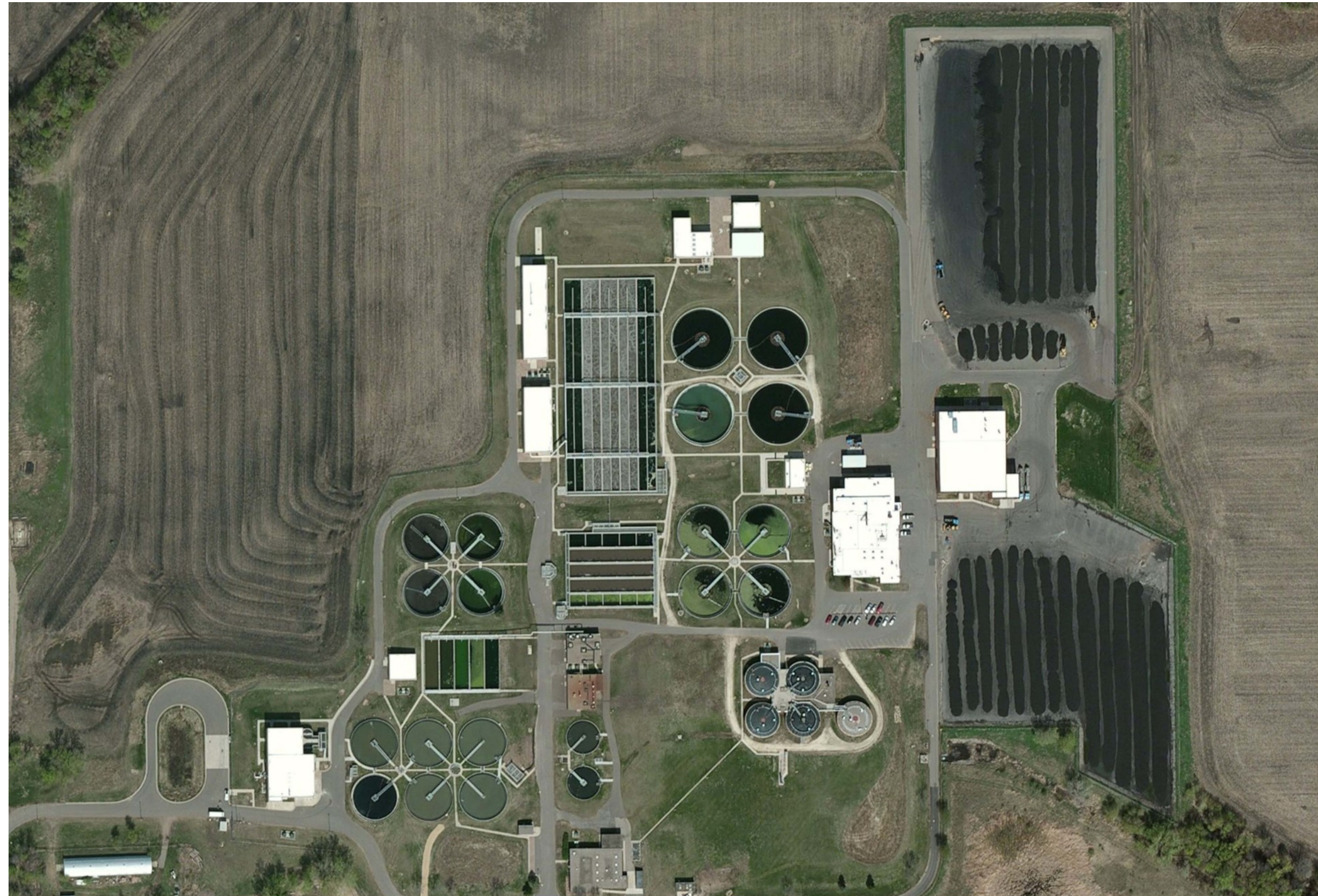
2005 - Solids Processing Capacity Expansion was Deferred
