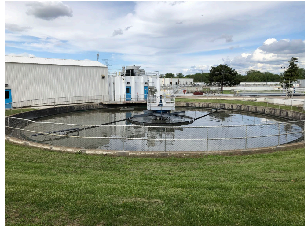
New Primary Clarifier Complex
