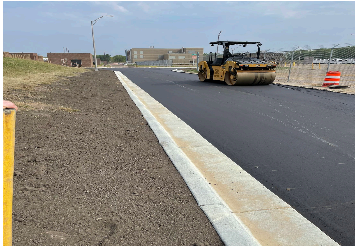
Civil / Site Work
