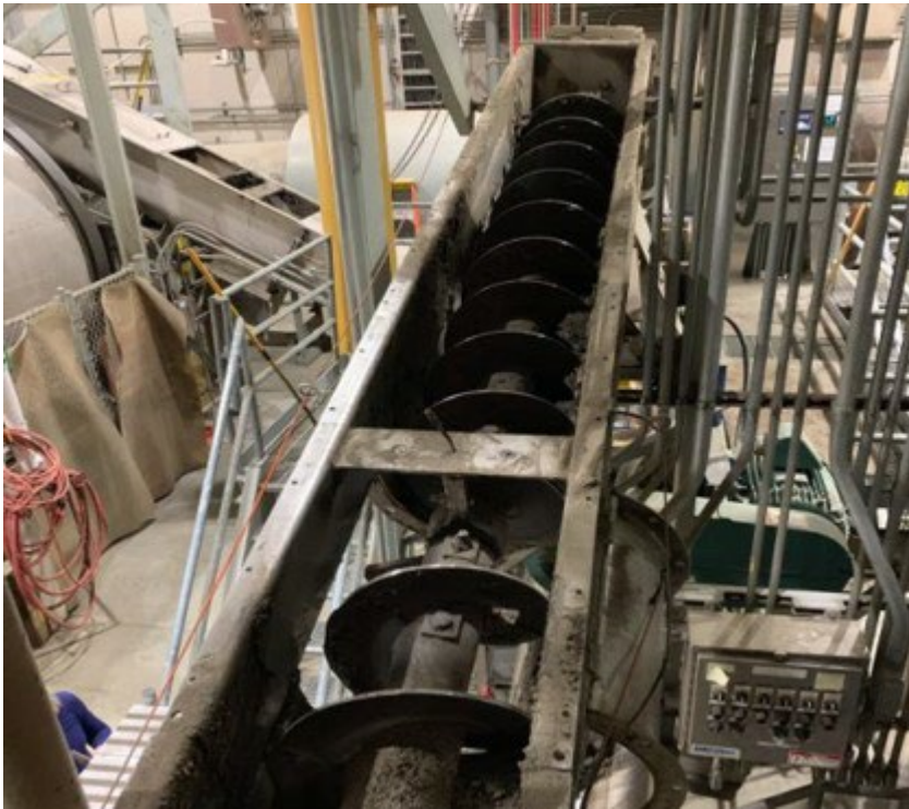
New Dryer & Existing Dryer Rehabilitation
