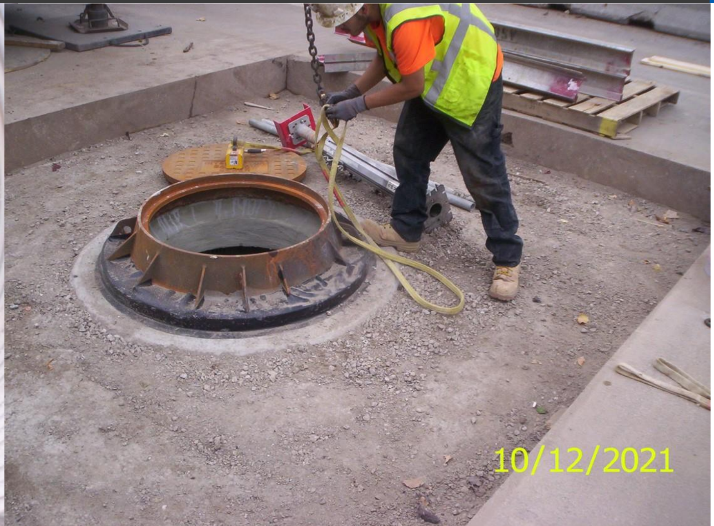
New top slab and casting are set to match existing street
