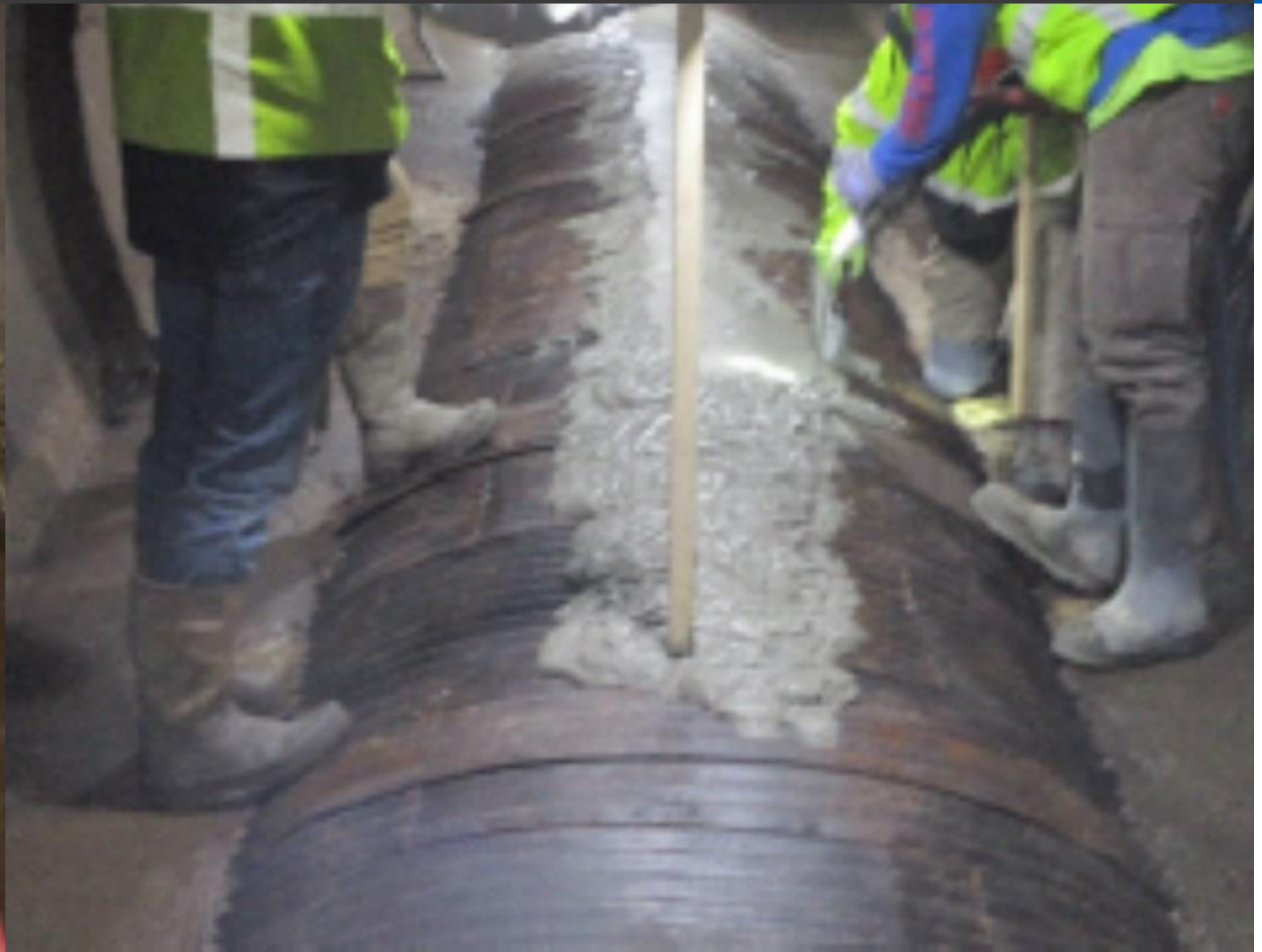
Geopolymer concrete mat is applied to corrugated pipe
