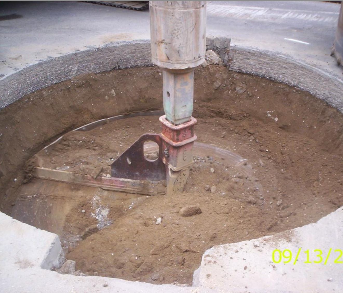
Excavations were drilled down to concrete sewer
