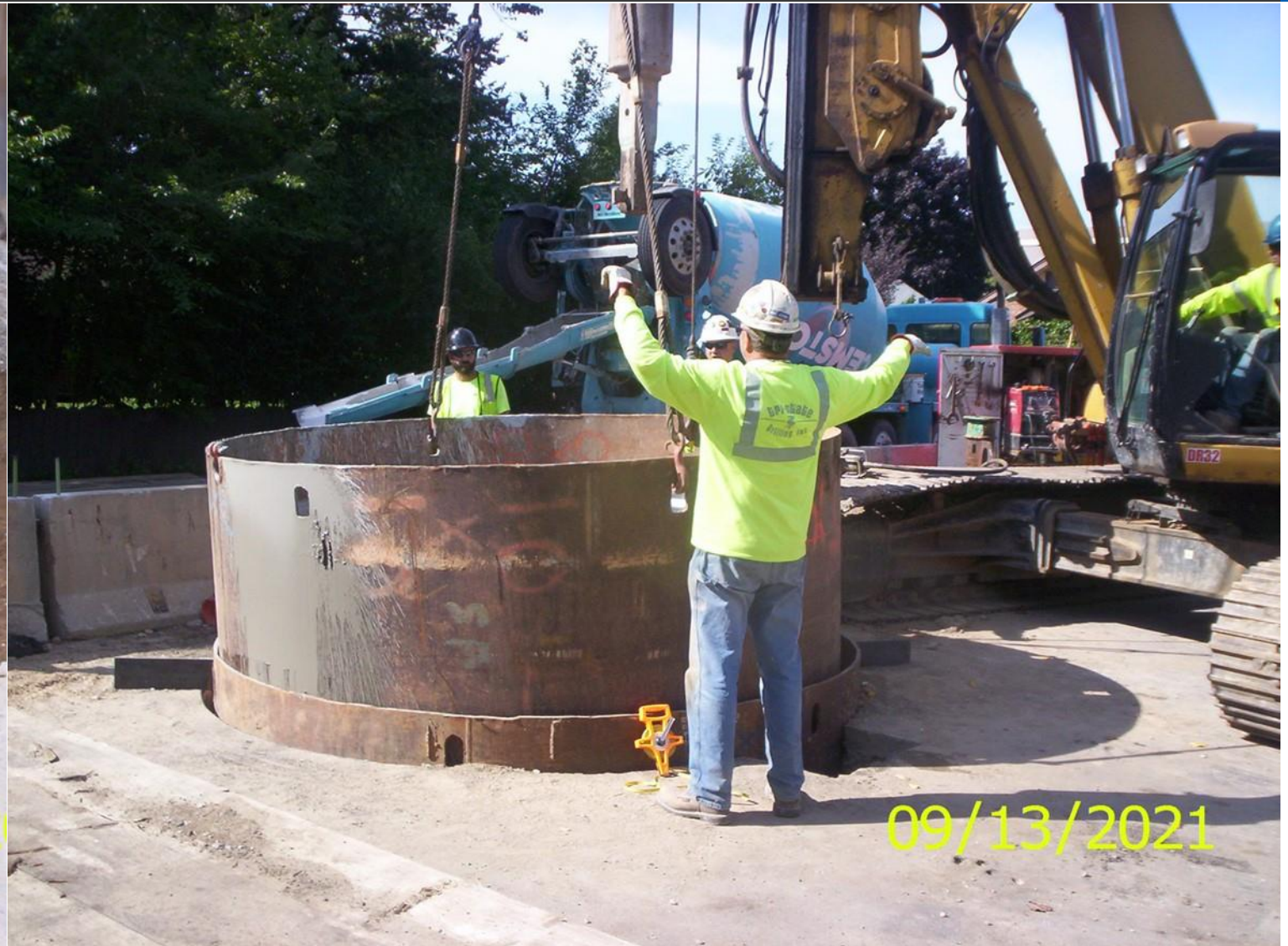
Steel casing was used to support the soils
