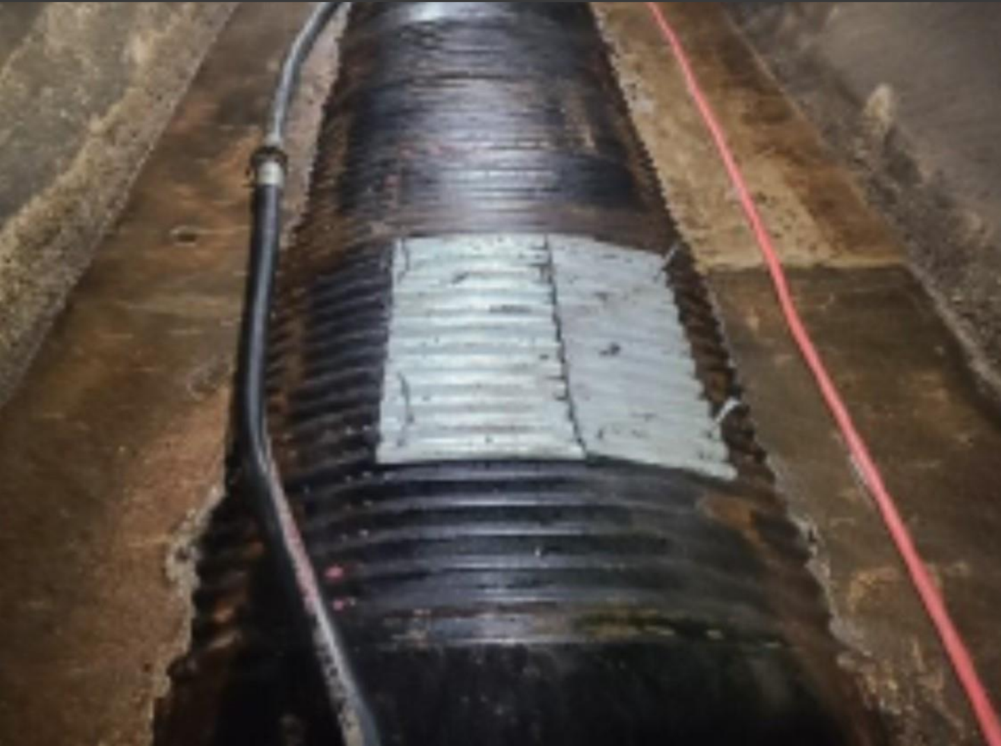
Interceptor pipe is repaired and cleaned
