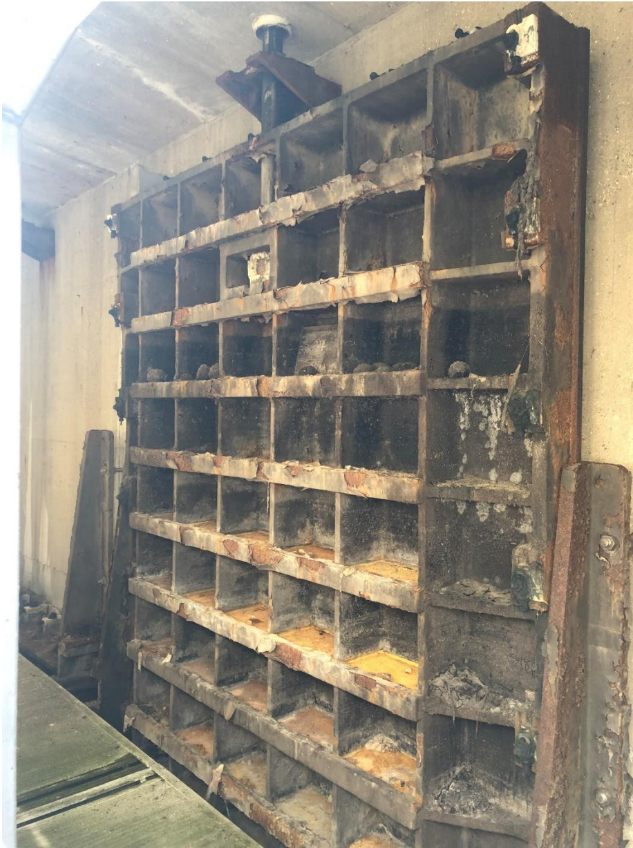
Existing Sluice Gate (2 @ 10' x10')
