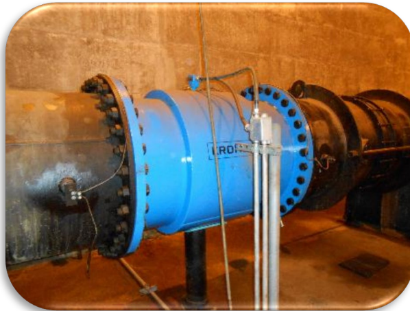
Magnetic flow meter on 36-inch Ductile Iron Pipe (Inverted Siphon)
